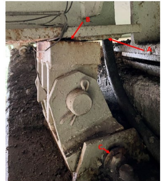
Example of emergency repairs on the Marsalis Bridge
