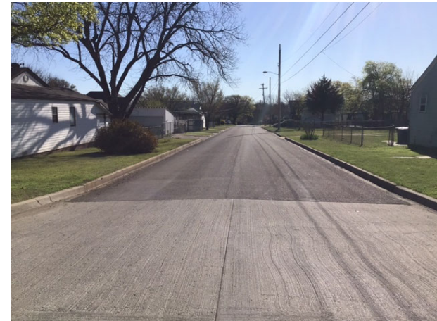
2900 8th Street—Microsurfacing Treatment
