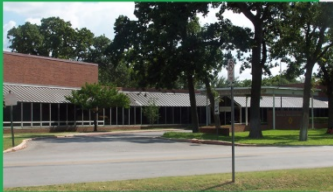
Bachman Recreation Center Interior Renovation
