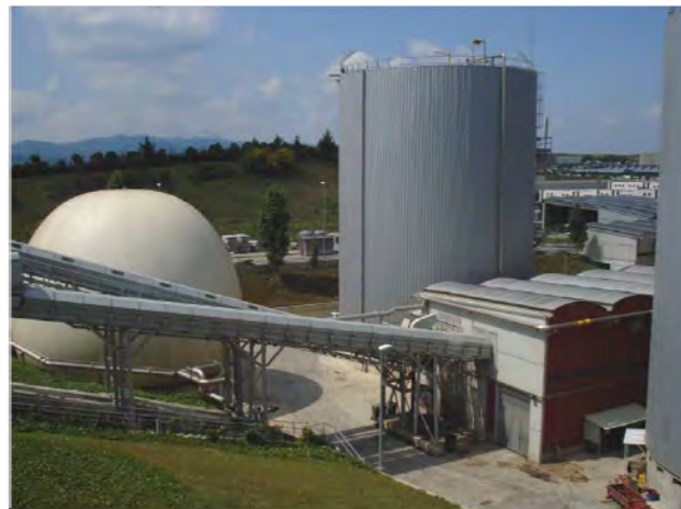
Figure 1 - Anaerobic Digestion Facility, Spain
