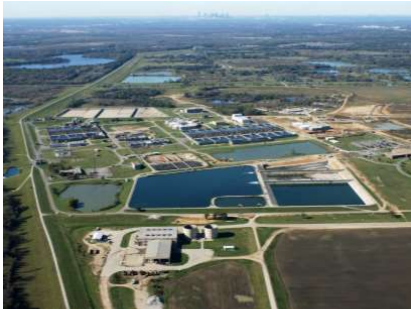
Figure 4-6: Southside Wastewater Treatment Plant
