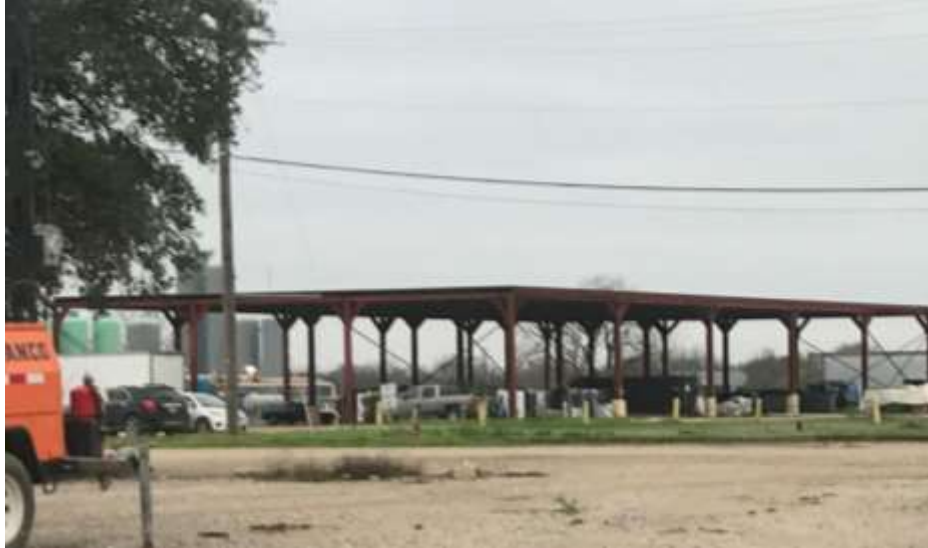
Figure E-20: CCRC Permanent Pole-Barn Structure
