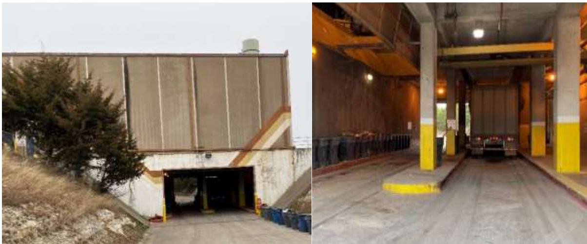
Figure C-19: Westmoreland Facility Transfer Trailer Truck Pull Through Location
