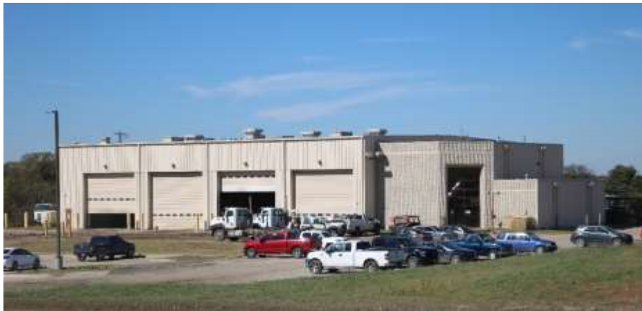
Figure E-3: Heavy Equipment Maintenance Shop
