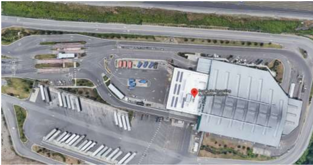
Figure 5-2: Bow Lake Recycling & Transfer Station
