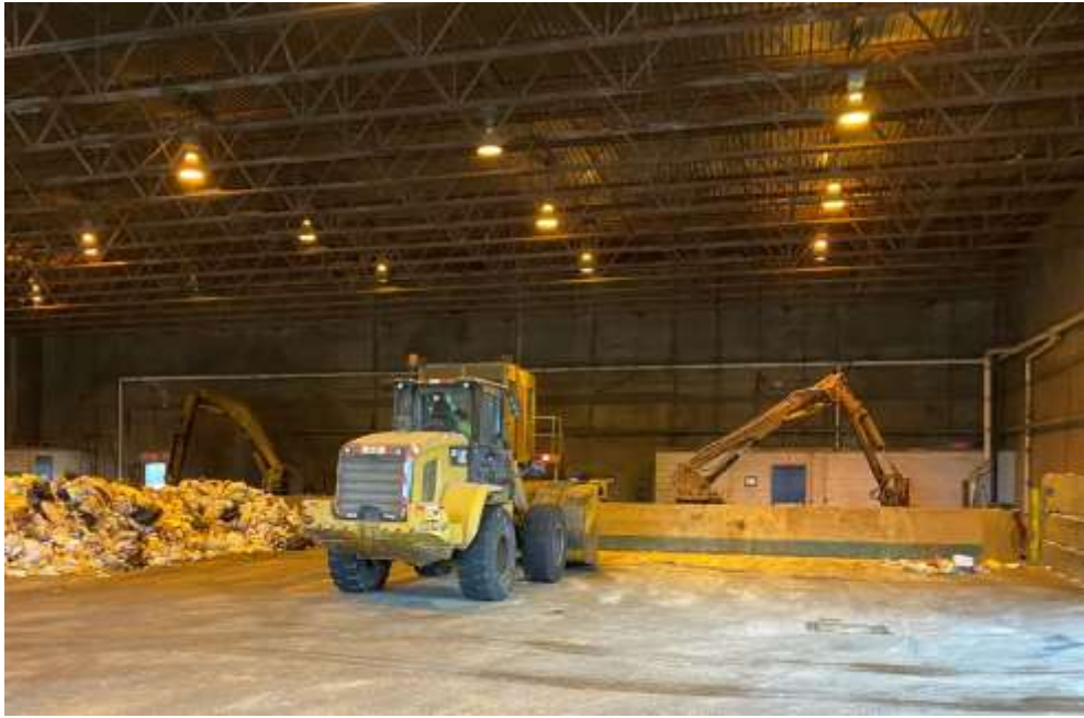
Figure C-18: Westmoreland Facility Hoppers
