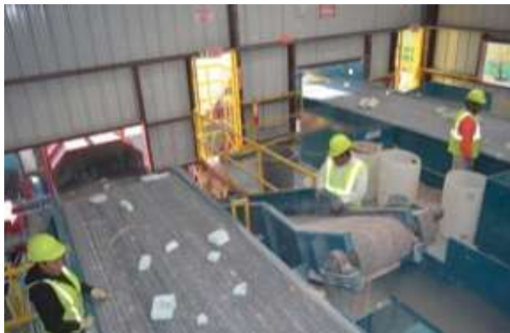
Figure 4-7: Champion Construction MRF Materials Processing Line
