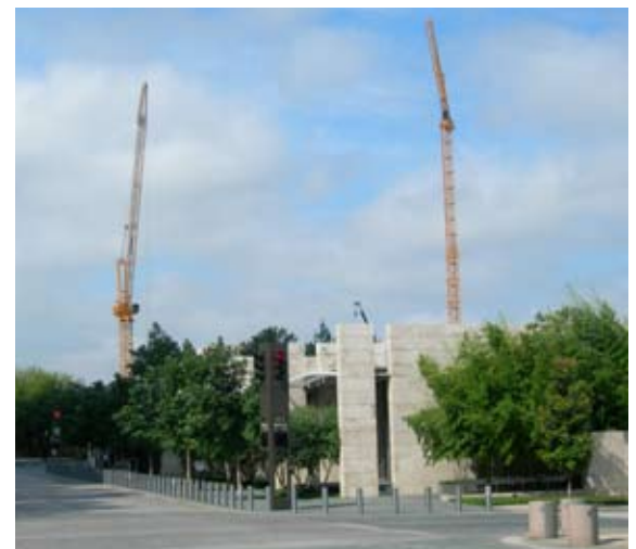
Cranes indicate construction activity near the Sculpture Garden.
