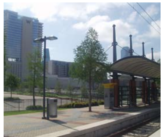
At many DART stations vacant land or underdeveloped land surrounds the station area indicating prime opportunities for new investment and development.
