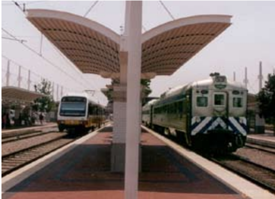
Utilizing both commuter and light rail technologies, DART and the City of Dallas have become a national leader in public transportation.
