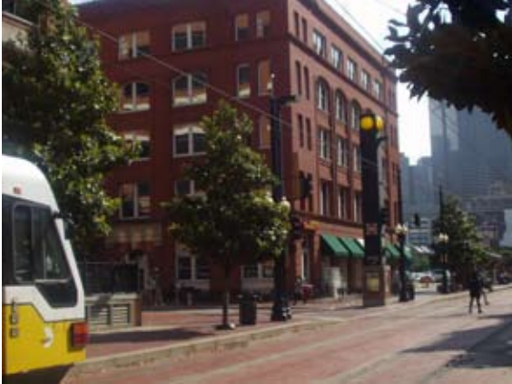
Developing Context Sensitive Design standards for DART stations will provide consistent standards that can be applied citywide.
