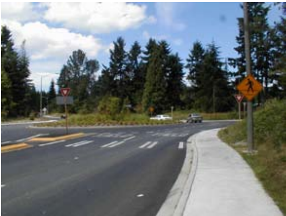
Traffic calming devices such as traffic circles and medians will help to reduce traffic speeds and enhance safety for pedestrians.
