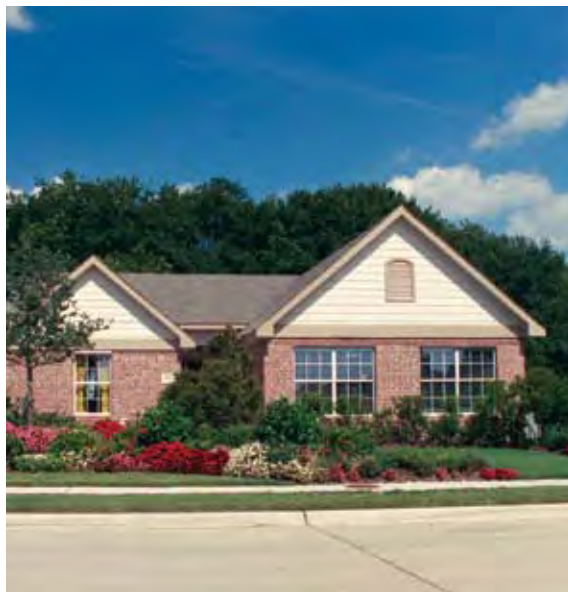
Single-family neighborhoods with detached houses like that above will remain an important part of Dallas' future.
