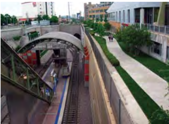
DART stations and multi-modal corridors will be characterized by high density mixed-use. Station areas will incorporate a range of uses and will be designed to fit within the communities in which they are located.
