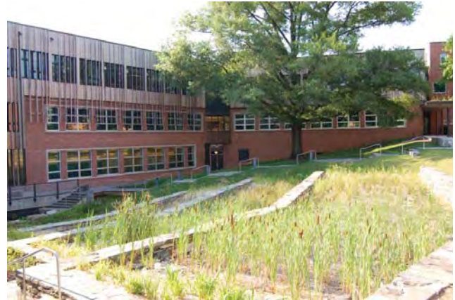
Wastewater is Treated On-Site in this Constructed Wetland in DC. Image Provided by Sidwell Friends School.
