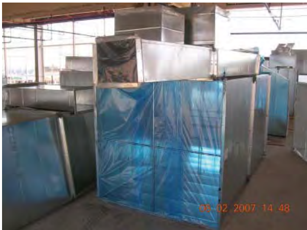
Sealed Ductwork.
