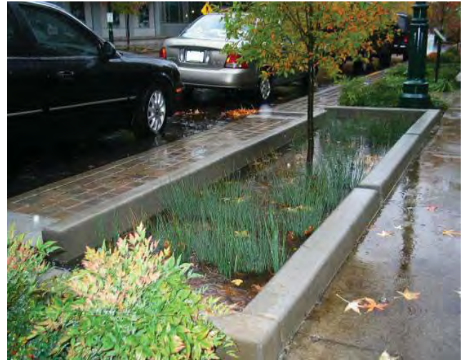
Sustainable Stormwater Strategy. Planter Collects Runoff to a Depth of 6 inches until it Flows back out into the Street and is Collected in the Next Downhill Planter.
