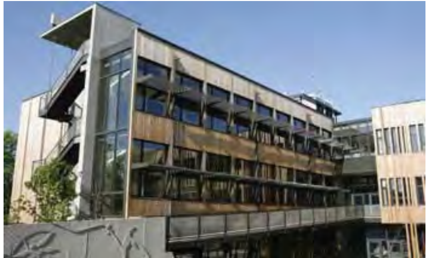
Horizontal Sun-shading Devices Protect Building Interior From Solar Heat Gain.
