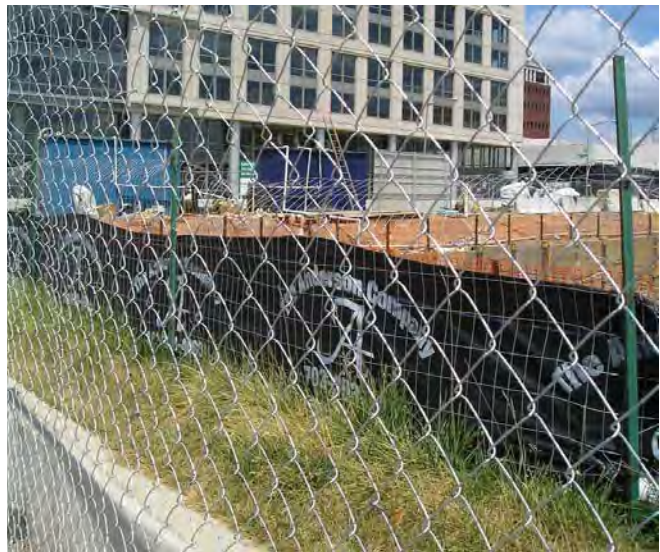
Erosion Control Strategy: Silt Fence.
