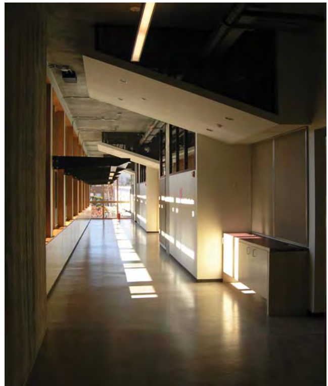
Interior Light Shelves and Clearstory Windows Bounce Daylight Further into Classroom Spaces.
