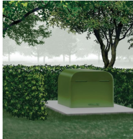
3. Allow a minimum of 10-foot access in front of a transformer and 5 feet around sides and back.
