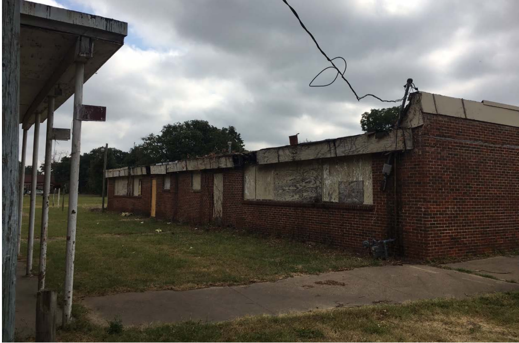
Separate classroom building for the lower grades.
