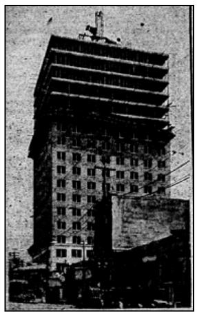
Figure 11. The Allen Building with brickwork completed to the fourteenth floor (*Dallas Morning News*, 7 March 1926:1).
