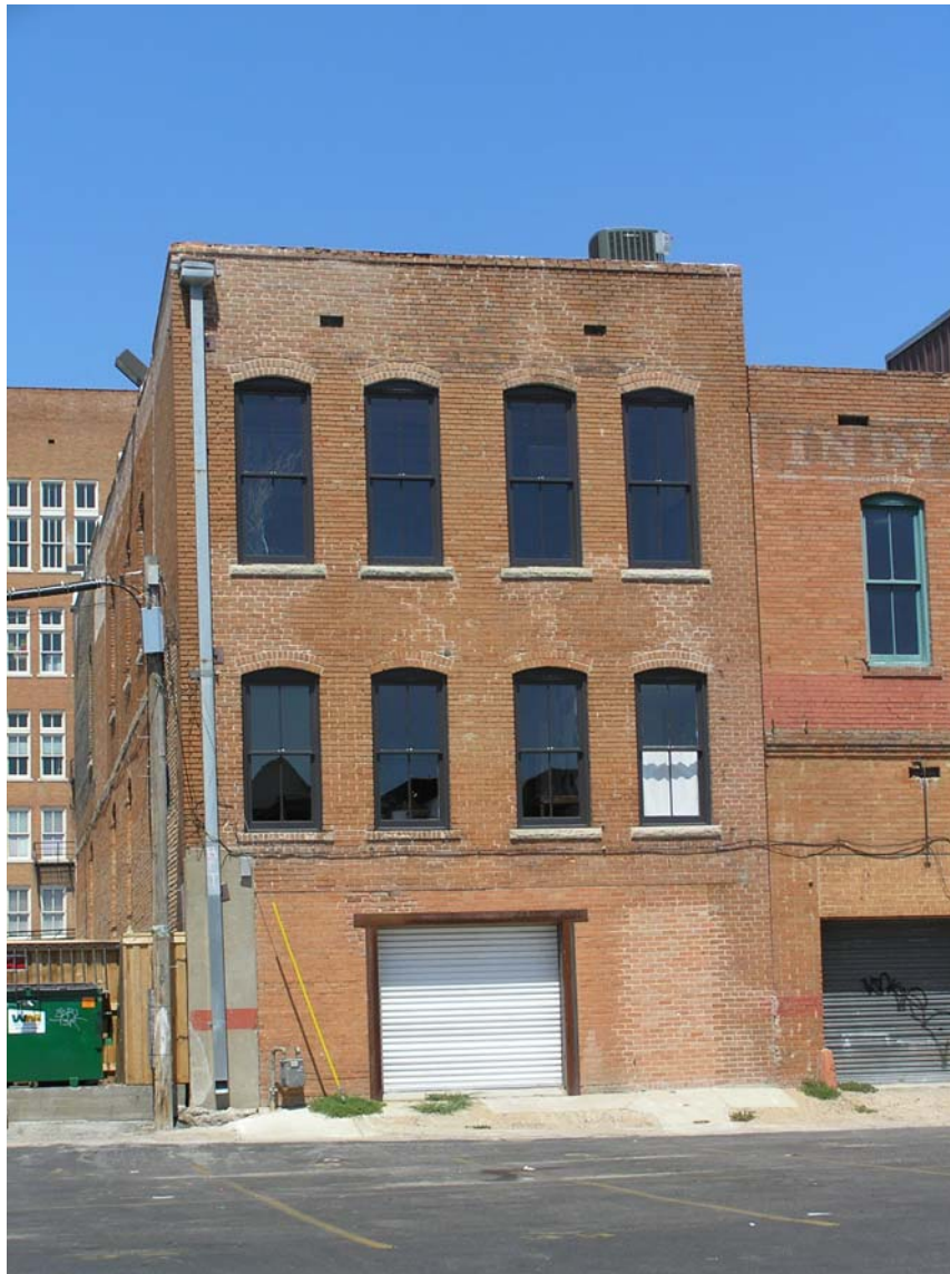
Bluitt Sanitarium Building – Photo #5. South Elevation Camera facing North 2036 Commerce Street, Dallas, Texas Marcel Quimby, photographer September 2005
