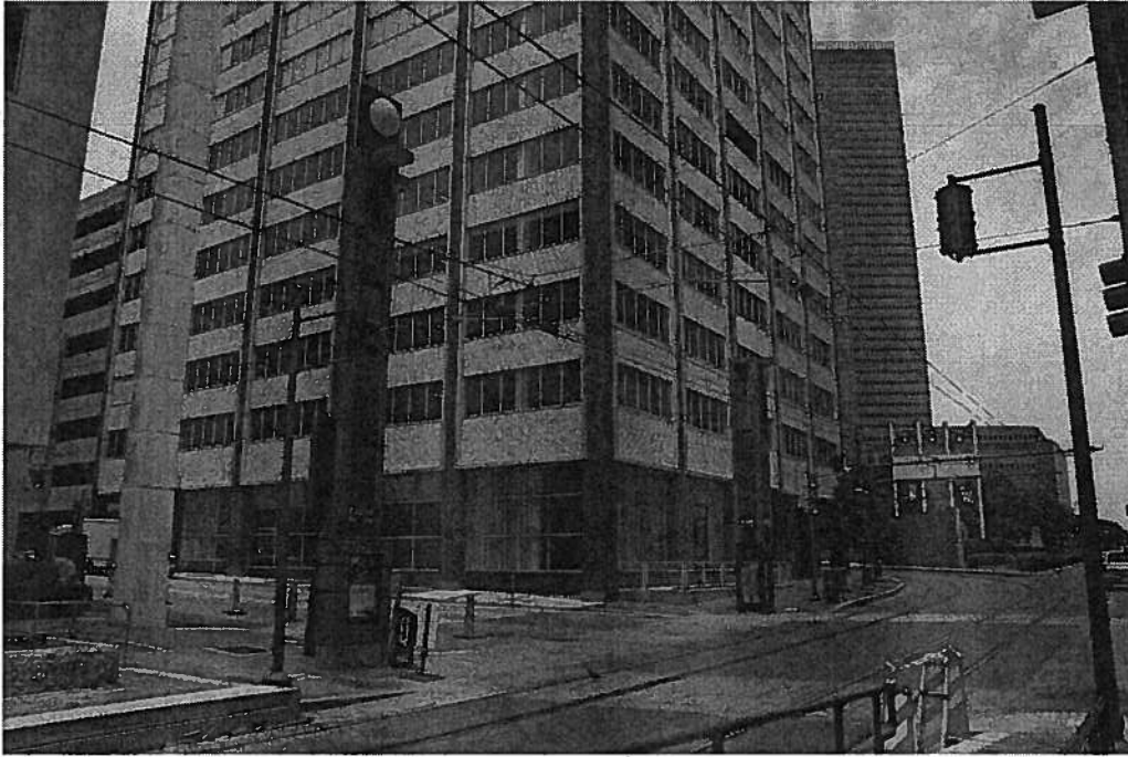
1960 Tower, ground floor, southwest oblique
