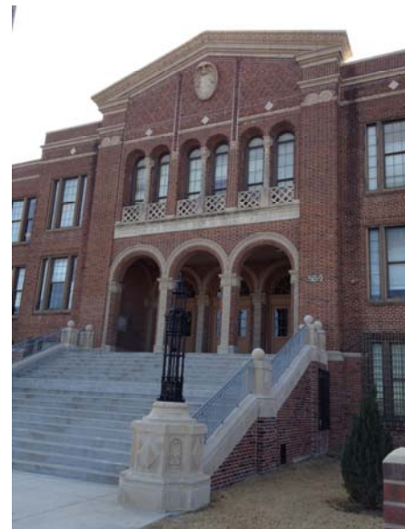
Front entry steps leading to loggia and front entrance.
