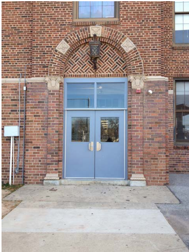
Detail of historic exterior door surround at west facade
