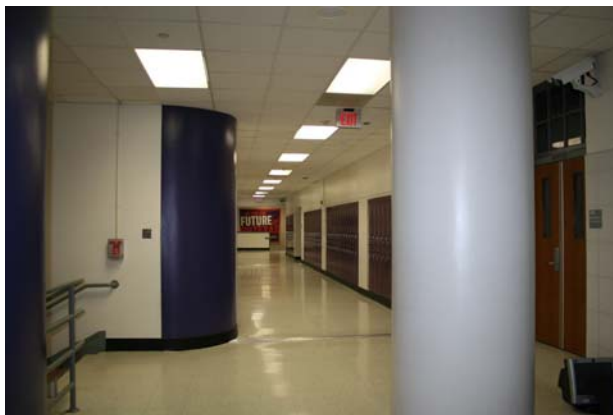
Third floor corridor with newer resilient tile floor, encased columns and 2' x 4' lay in ceiling.
