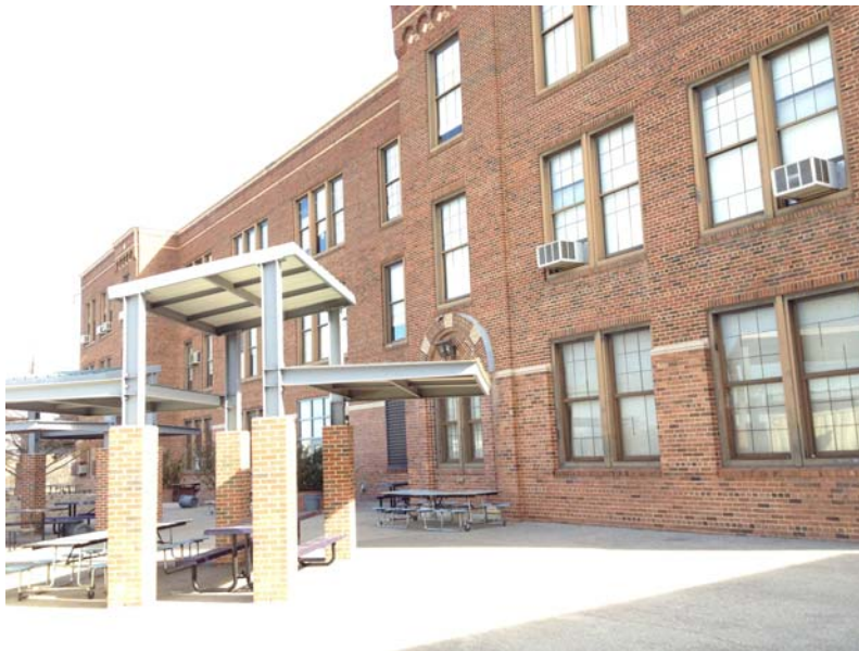
West facade, with brick and metal picnic shelters at adjacent patio.
