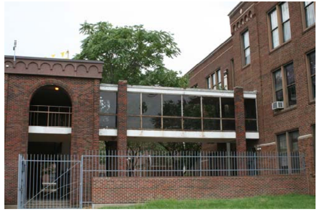
North facade of Science Addition at right (1963).
