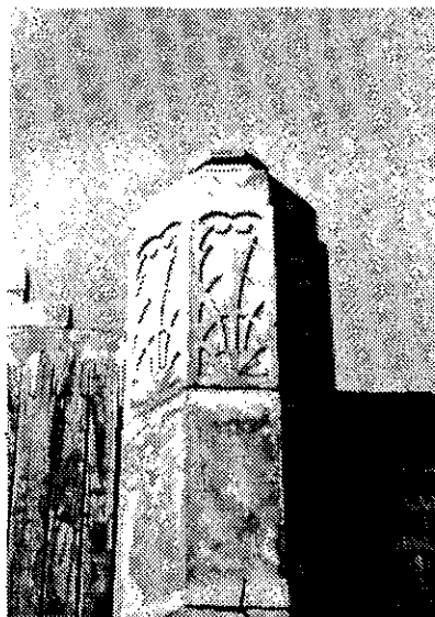
BELOW: Dewitt & 3rd.
