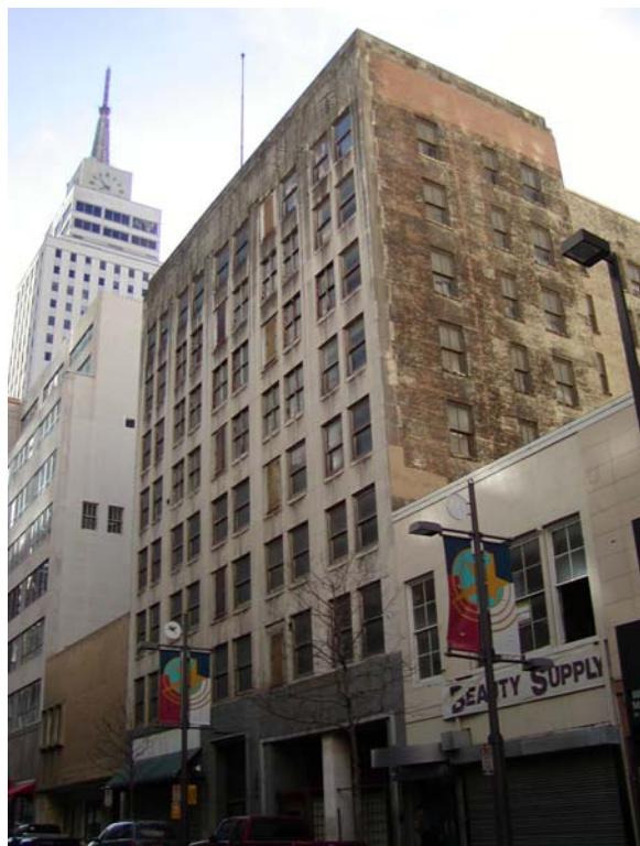
Sumpter Building (1913) 1604 Main Street
