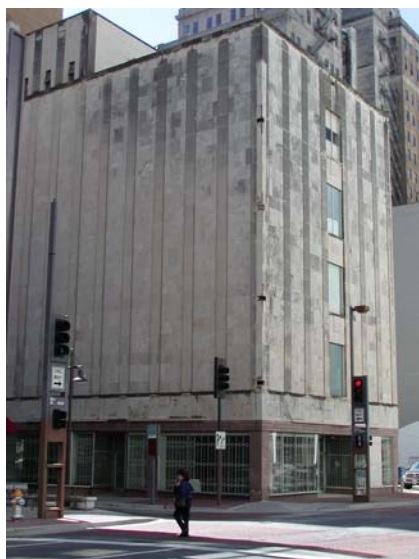
Original building, c. 1955 – 2005
