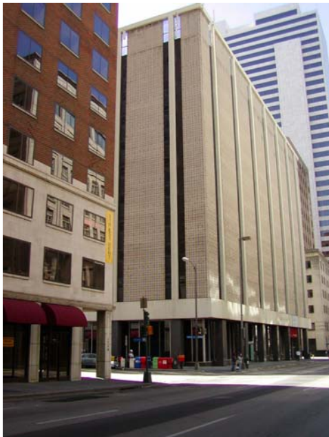
Neiman Marcus Parking Garage (Dal-Park Garage; 1968) 1600 block of Commerce Street
