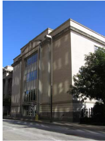
Activities Building Addition (at west) Photographer: Marcel Quimby, October 27-29, 2007.
