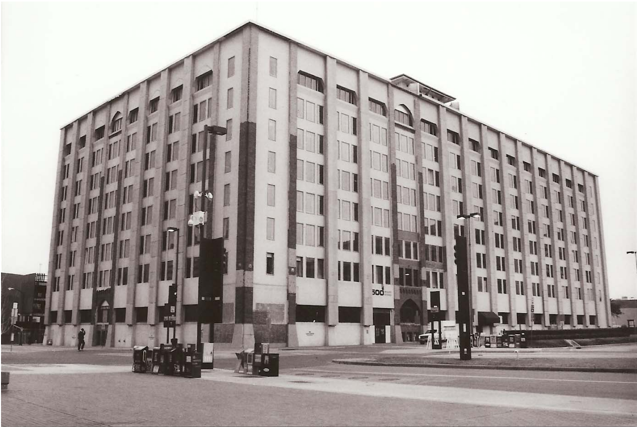
Photo 3: Butler Building; Intersection at South Ervay Street and Marilla Street, looking south-east to the Butler Building. Camera facing South-East.
