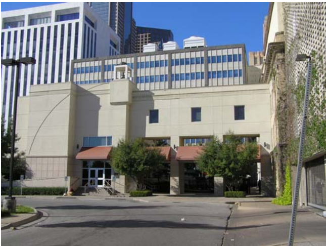
New 'link' between Activities building and 1818 Wood, viewed from the south. Photographer: Marcel Quimby, October 27-29, 2007.
