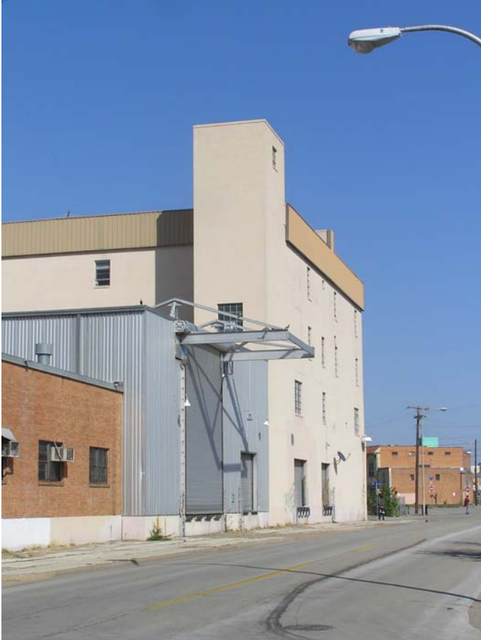
Photograph 12: Marilla Street from intersection at St. Paul Street. DP&L Distribution Headquarters at left. Camera facing Northeast.
