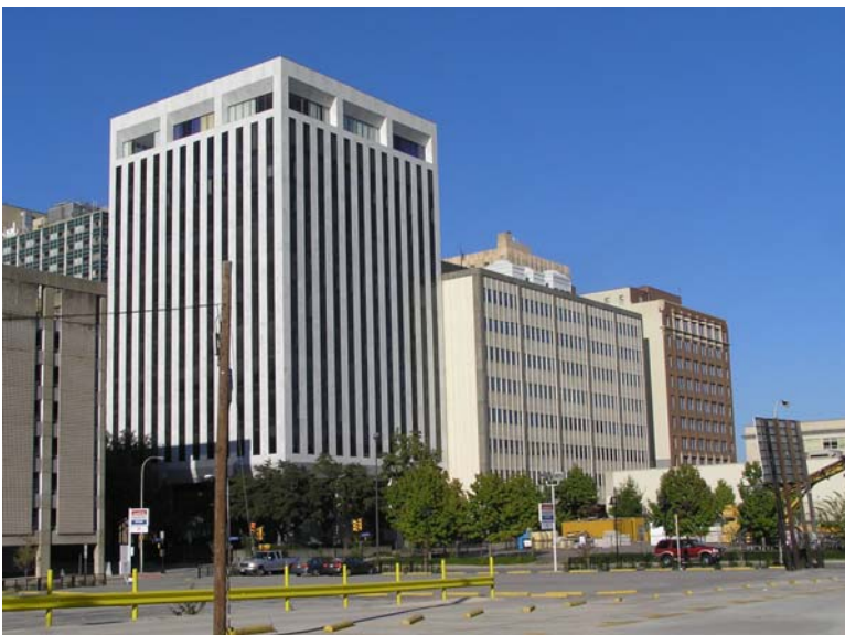
Photograph 9: Wood Street from parking lot just north of Young Street. Camera facing northeast.
