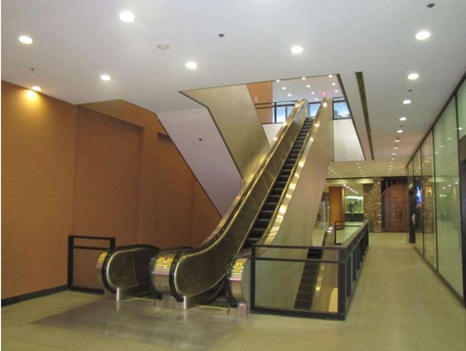
TX_Dallas County_One Main Place_0017 East escalator group at plaza level – camera facing northwest
