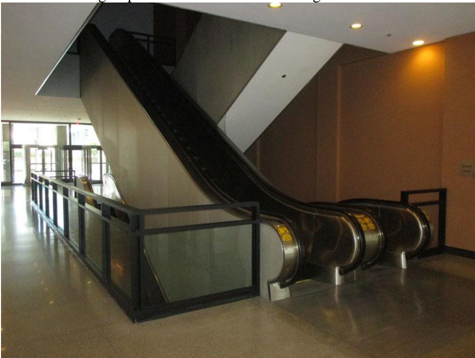
TX_Dallas County_One Main Place_0014 West escalator group at first floor – camera facing northeast
