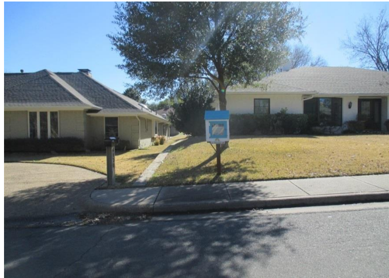
located too close to adjacent property line
