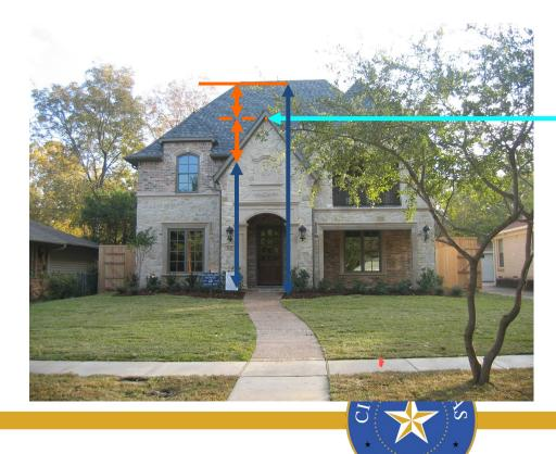
Height is a horizontal plane measured ½ way between peak and eave.
