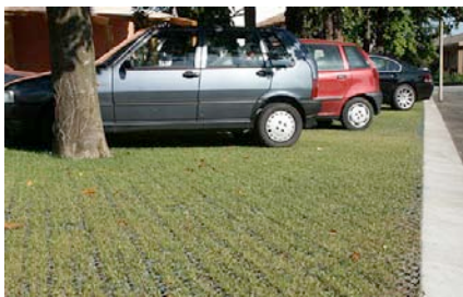
Pervious structure supporting growth of grass
