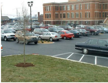
Porous asphalt parking lot
