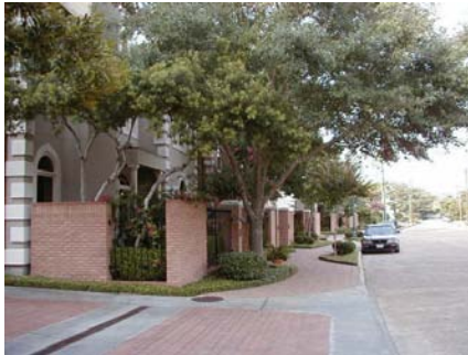
Pervious brick pavers on sidewalks and driveways
