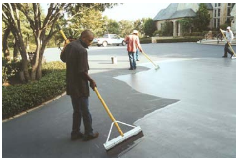
Seal coating as surface maintenance
