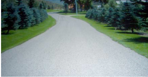
Figure 11. Chip Seal Overlay with Reflective Aggregate
