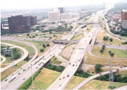
Dallas freeway interchange
