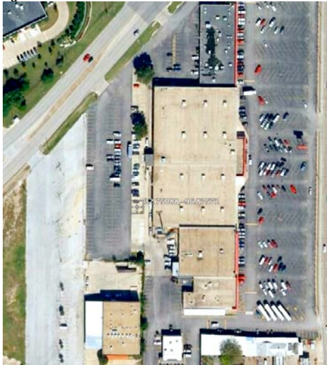
Figure 3. Dallas commercial site
