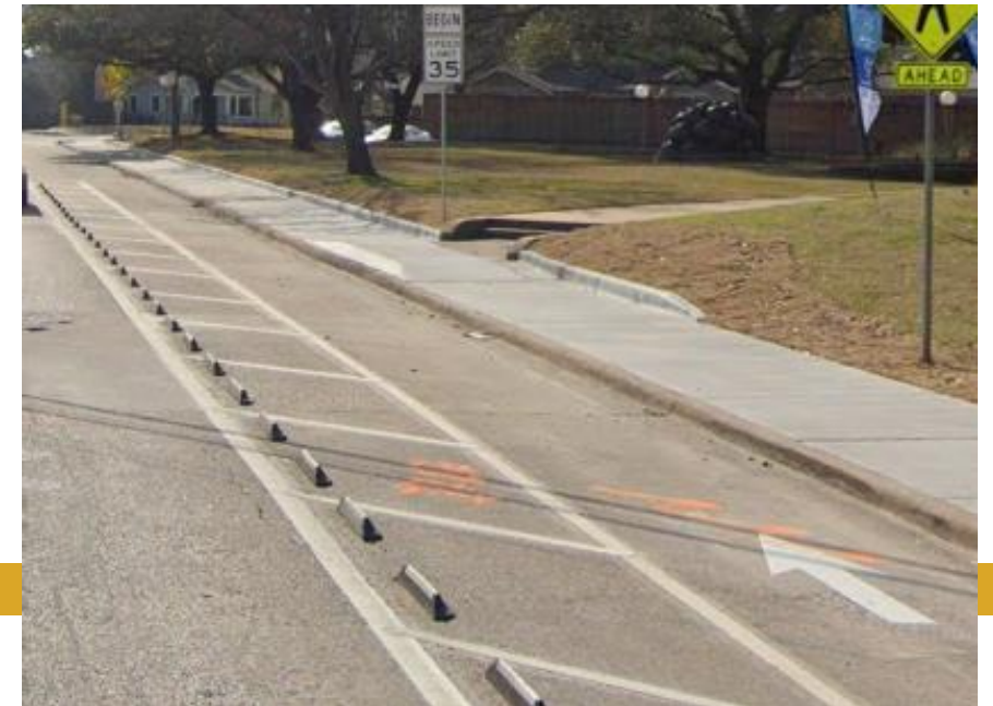
Abrams Ave: project has been successful
