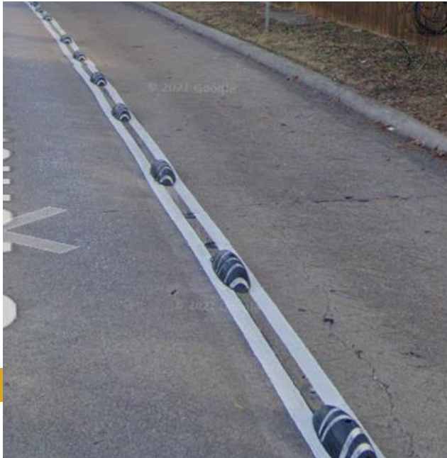
Vernon Ave: newly installed
