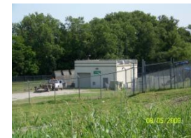
Rochester 4 pumps – 122,256,000 GPD Cole Park 4 pumps – 129,600,000 GPD
