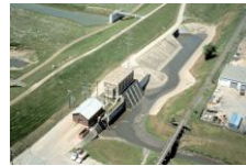
Baker (drainage area - 3,418 acres) 15 pumps – 1,900,800,000 GPD
