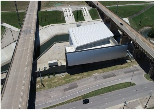
Able Pump Station
