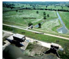
Hampton (drainage area - 6,355 acres) 11 pumps – 876,240,000 GPD
