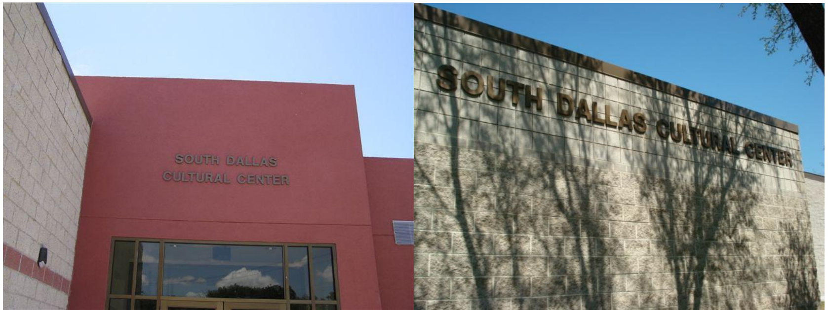
Exterior views of South Dallas Cultural Center
