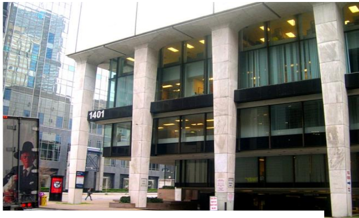
Corner of Elm and Field Street - Existing
