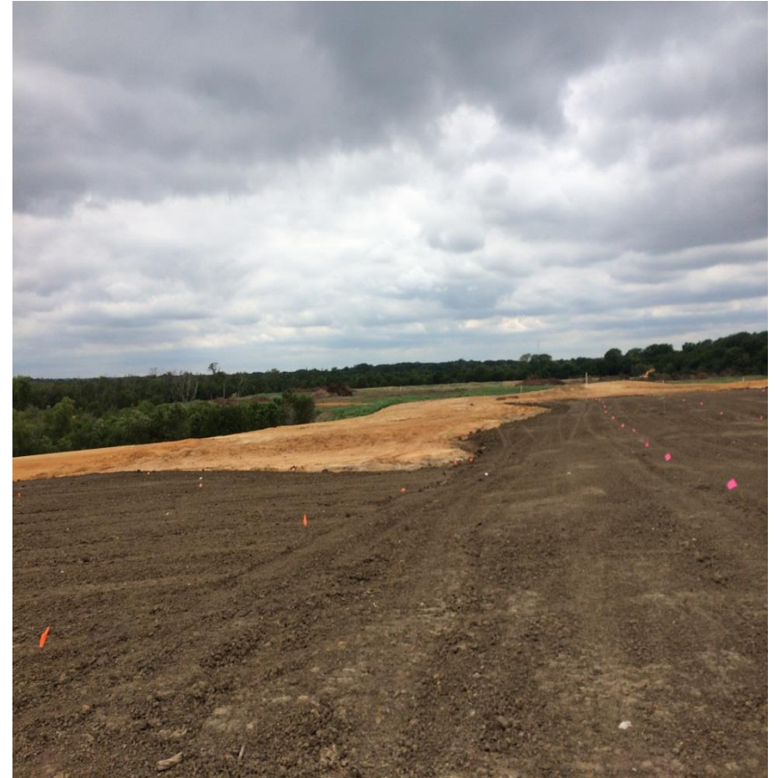
Cap Repair with Clay & Vegetative Support
