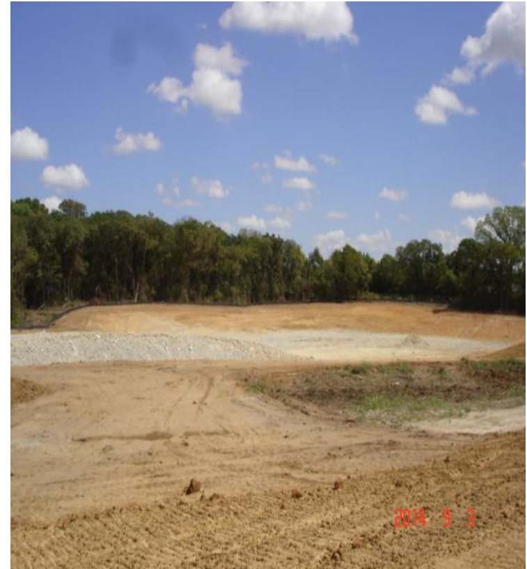
Borrow Area "C"
