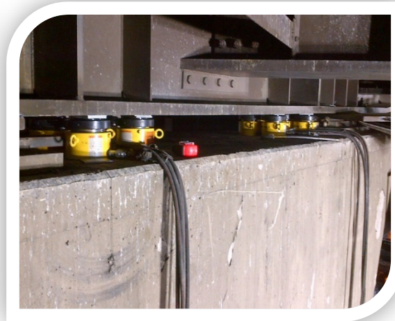
JACKING OPERATION AT INWOOD BRIDGE
