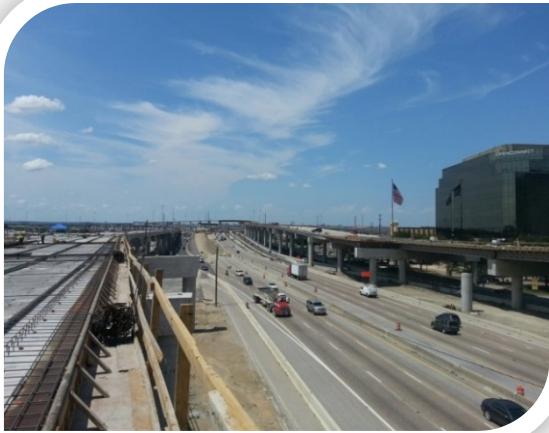
IH 635 LOOKING WEST FROM ANAHEIM RD.
