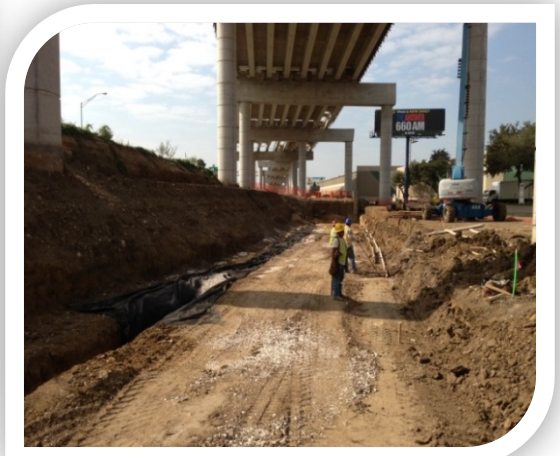
BRIDGE 7C AND MSE WALL 4 SB LOOP 12
