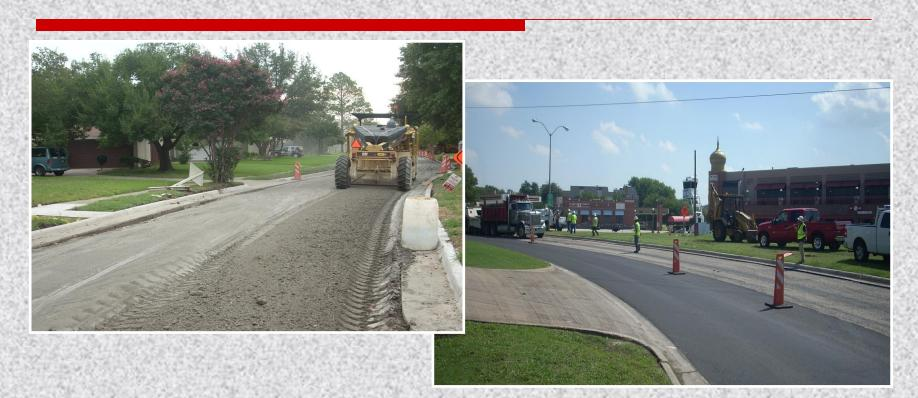
**Re-Surfacing** – This treatment removes the entire asphalt surface, and pulverizes and recycles the old material with new asphalt binder. The new asphalt surface is then placed over the entire surface, compacted, and smoothed to a proper finish. Curb and gutter repair, if needed, is accomplished with the re-surfacing efforts. **Cost:** \$200K per lane-mile. Life: 15-20 years (with maintenance).
