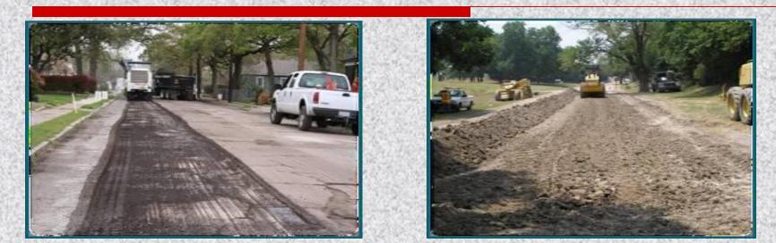
**Rehabilitation** - A treatment for ASPHALT STREETS when a large portion of the surface and the base have deteriorated to an unsatisfactory level. It includes the full-depth repair of base failures, followed by a chip seal, and a new two-inch layer of hot mix asphalt placed over the entire treated segment. Candidate streets are predominately residential asphalt surfaced streets without curb and gutter. **Cost:** \$160K per lane-mile. **Life:** 10-12 years.
