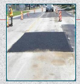
**Slurry Seal** - This treatment for CONCRETE STREETS WITH ASPHALT SURFACE consists of a ¼-inch layer of sand and fine stone mixed with asphalt emulsion. This seals and smooths the surface and conceals scars from previous repairs. It is used predominately for residential roads with curb and gutter. The work is outsourced to a specialized contractor – after Street Services performs preparation work (such as minor base repair and crack sealing). **Cost:** \$13K per lane-mile. Life: 5-7 years.
