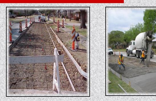
**Partial Reconstruction** - This is a method used on CONCRETE STREETS. It is **removal and replacement of large, failed sections**, including breakout and removal of old pavement, repair of any base failures, and placing new concrete. To be a candidate for this repair, residential and thoroughfare streets must have less than 25% of failed area.
