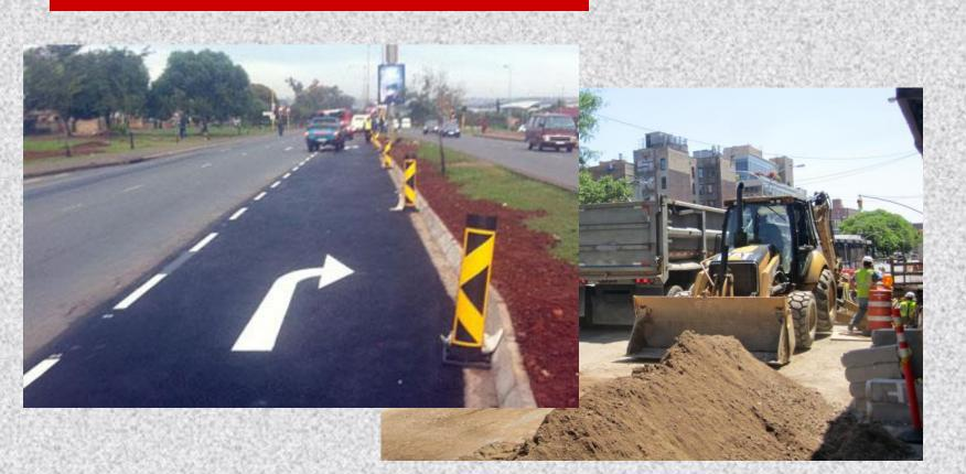
Street and alley repairs by the Dallas Water Utilities are associated with pipeline replacement. For asphalt streets the City policy requires that an entire lane be reconstructed at the location for where the pipeline is replaced. From joint to joint for concrete streets.
