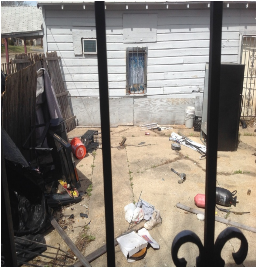
Illegal Outside Storage, Litter and Substandard Structure
