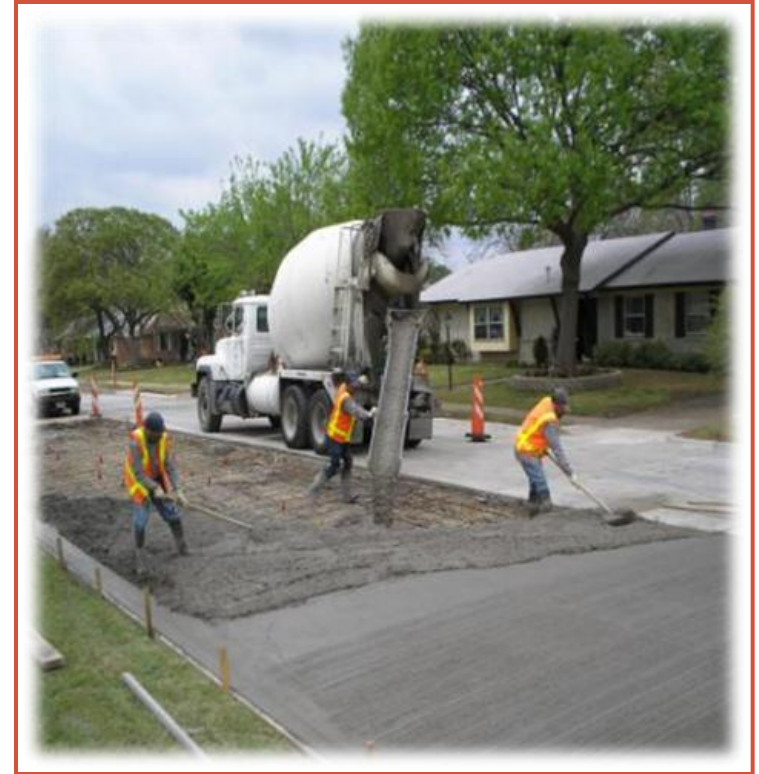
Concrete Partial Reconstruction for "C" rated (and some "D" rated) streets
