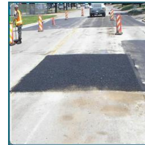
Full-Depth Asphalt Repair for "C" rated streets
