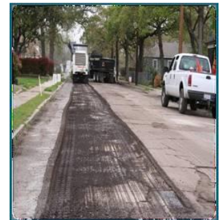
Asphalt Rehabilitation for "D" rated streets
