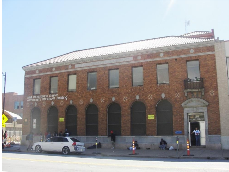
1822 Young Street Otis Elevator Building 1922 Current Owner: First Presbyterian Church Institutional
