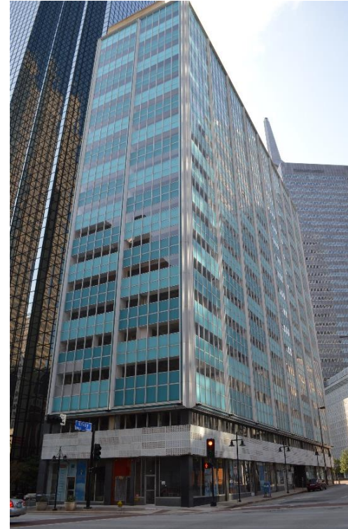
211 N Ervay 1958 Current Owner: Alterra 211 North Ervay LLC Office/retail – under construction City Center TIF ($2,000,000)
