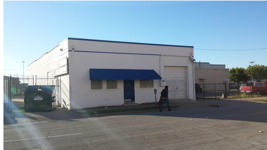
1808 Canton Street Warehouse 1935 Current Owner: William L. Smith Sr & ET AL
