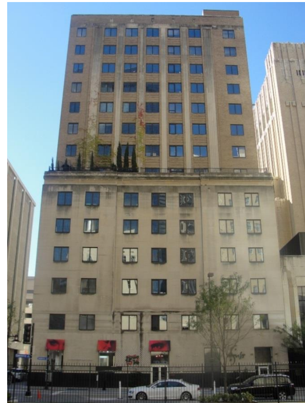
1512 Commerce Street Continental Supply/Texaco Building 1903 (later additions) Current Owner: DPL Loans Holdings LLC Residential/retail City Center TIF and Federal Tax credit
