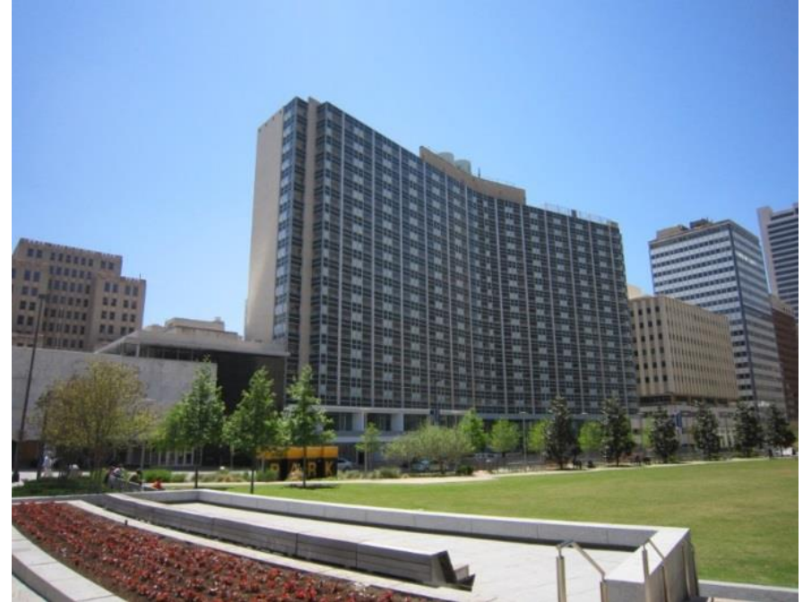
1914 Commerce Street Statler Hilton Hotel 1956 Current Owner: Commerce Statler Development LLC Vacant – under construction Downtown Connection TIF ($46,500,000 - combined with Old Public Library) and Pending Federal Tax Credit – Future construction
