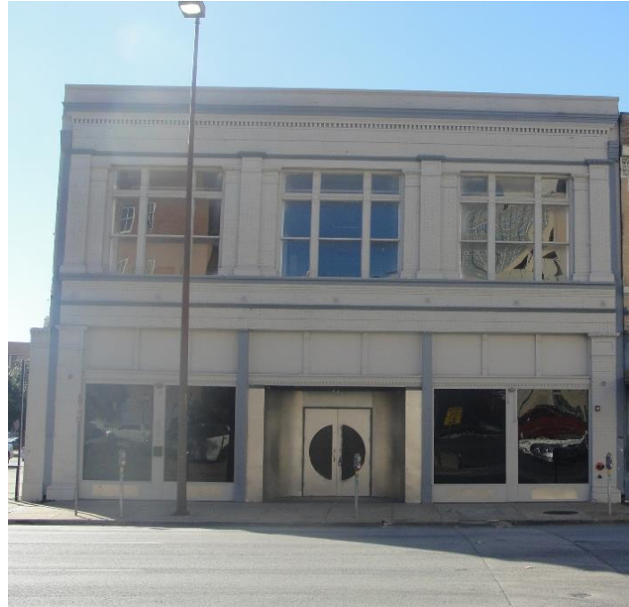
2026 Commerce Street Two-story commercial building c. 1915 Current Owner: CADG 2026 Commerce LLC Vacant
