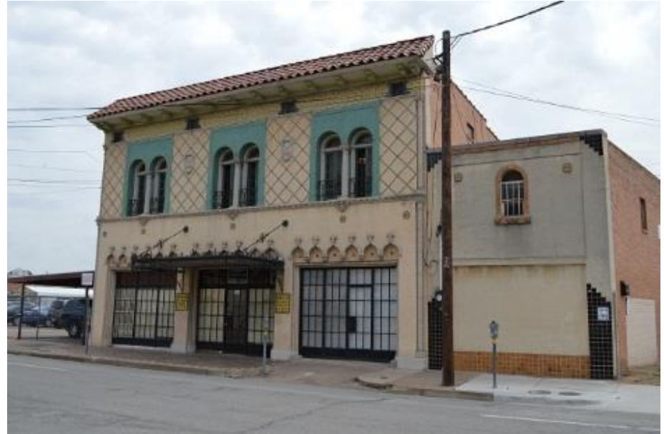
1908 Canton Street (1907 Marilla Street) Desco Tile Company Building c. 1923 Current Owner: Amigos Pottery Inc Office/retail
