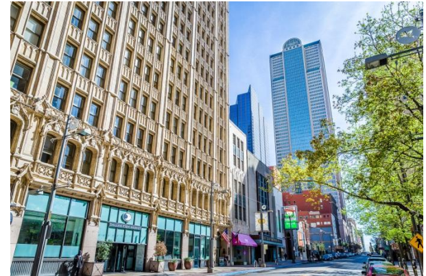
Storefronts, streets, sidewalks, awnings, landscape, and variety in scale: the historic and authentic urban fabric of Main Street. Thomas Garza Photography, courtesy of Downtown Dallas, Inc
