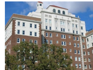
Lake Cliff Tower
