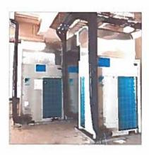
28 high energy efficient VRV HVAC units are installed
