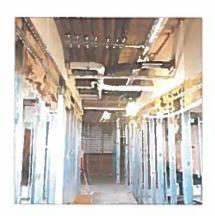
Dry wall, insulation, and fire tape at ceiling is completed on 17 apartment floors
