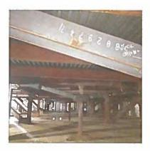
New structural support steel was fabricated and it is installed on levels 6-7 (pictured level 7)
