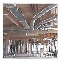
Mechanical rough – ductwork is installed on 12 apartment floors
