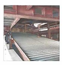
Floor cutouts were made and new steel ramps are installed from the street level to the added parking garage on fl. 6-8 (behind the windowless marble façade)
