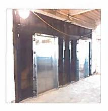
Elevator openings were cleared and new frames, sills and doors are installed on 15 floors
