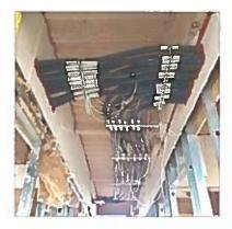
Mechanical rough - refrigerant piping is installed on 12 apartment floors
