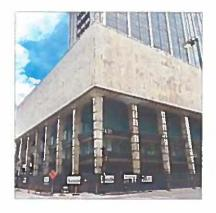
94% of the historic marble is removed. THC / NPS approved the refurbished marble mock installation (seen on the 3rd from right column crown)
