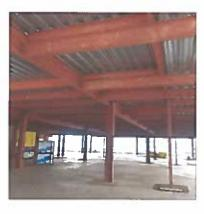
New steel structure installed on fl. 9 (amenity deck) & 10 (above)
