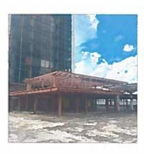
New steel structure is installed for restaurants and bars on the 75,000 sq.ft. amenity deck
