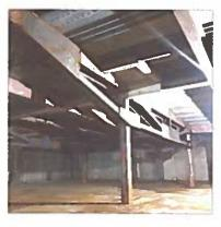
New structural support steel was fabricated and it is installed on levels 6–7 (pictured level 6)
