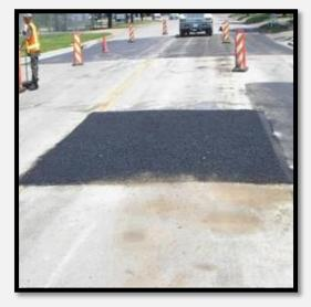
**Slurry Seal** - This treatment for CONCRETE STREETS WITH ASPHALT SURFACE consists of a ¼-inch layer of sand and fine stone mixed with asphalt emulsion. This seals and smooths the surface and conceals scars from previous repairs. It is used predominately for residential roads with curb and gutter. The work is outsourced to a specialized contractor – after Street Services performs preparation work (such as minor base repair and crack sealing). **Cost:** \$13K per lane-mile. **Life:** 5-7 years.
