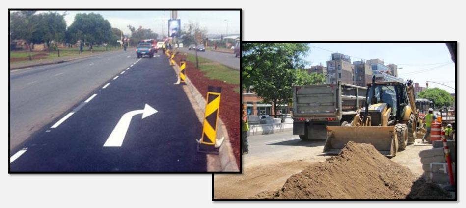
Street and alley repairs by the Dallas Water Utilities are associated with pipeline replacement. For <u>asphalt streets the City policy requires that an entire lane be reconstructed at the location</u> for where the pipeline is replaced. From joint to joint for concrete streets.
