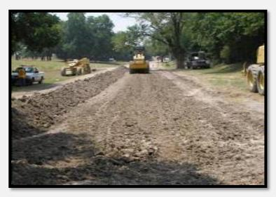
**Rehabilitation** - A treatment for ASPHALT STREETS when a large portion of the surface and the base have deteriorated to an unsatisfactory level. It includes the full-depth repair of base failures, followed by a chip seal, and a new two-inch layer of hot mix asphalt placed over the entire treated segment. Candidate streets are predominately residential asphalt surfaced streets without curb and gutter. **Cost:** \$150K per lane-mile. **Life:** 10-12 years.
