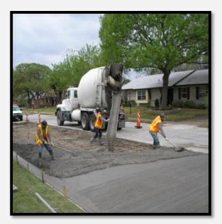
**Partial Reconstruction** - This is a method used on CONCRETE STREETS. It is **removal and replacement of large, failed sections**, including breakout and removal of old pavement, repair of any base failures, and placing new concrete. To be a candidate for this repair, residential and thoroughfare streets must have less than 25% of failed area.
