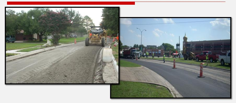
**Re-Surfacing** – This treatment removes the entire asphalt surface, and pulverizes and recycles the old material with new asphalt binder. The new asphalt surface is then placed over the entire surface, compacted, and smoothed to a proper finish. Curb and gutter repair, if needed, is accomplished with the re-surfacing efforts. **Cost:** \$245K per lane-mile. Life: 15-20 years (with maintenance).
