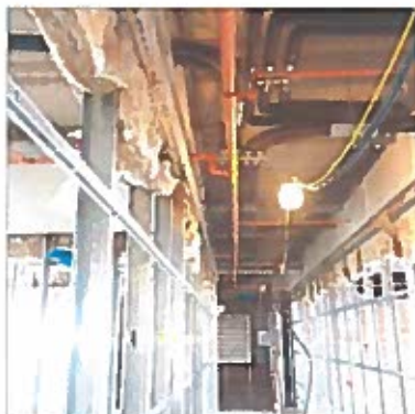
Fire sprinkler rough-in is installed on 7 apartment floors
