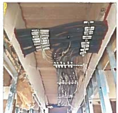
Mechanical rough - refrigerant piping is installed on 12 apartment floors
