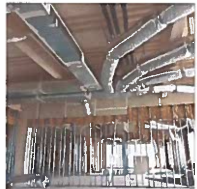
Mechanical rough - ductwork is installed on 12 apartment floors
