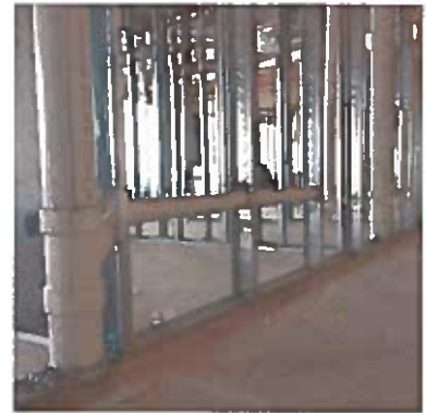
Plumbing rough is installed and completed on 12 apartment floors
