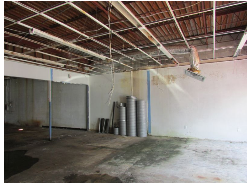
Deferred maintenance – vacant space
