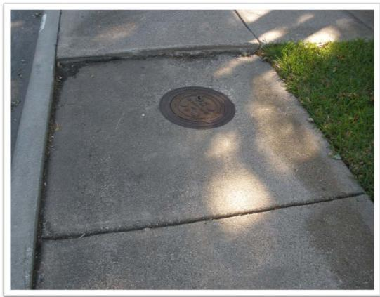
Sunken sidewalk around water meters is typically a result of poor soil compaction prior to sidewalk construction by the agent of the original home builder.
