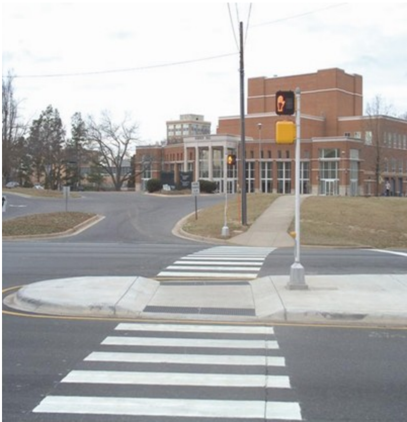
FIGURE 10: PEDESTRIAN REFUGE ISLAND AT INTERSECTION (SOURCE: FHWA)
