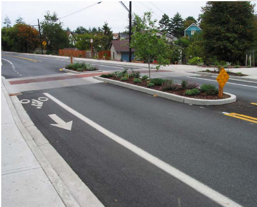
FIGURE 9: MID-BLOCK PEDESTRIAN REFUGE ISLAND
