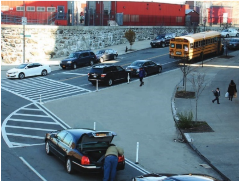
FIGURE 6 CURB EXTENSIONS USING ASPHALT TREATMENT, BOLLARDS:
