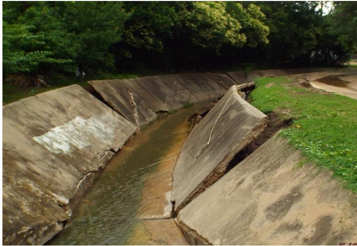
Channel at 3132 Silverton
