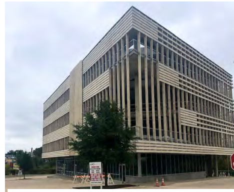
Construction of BookMark Center retail and office space as part of Half Price Books’ multi-phased development is nearly complete and available for lease.
