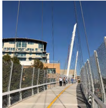
The Mockingbird Bridge opened for bikes and pedestrians in November 2017.
