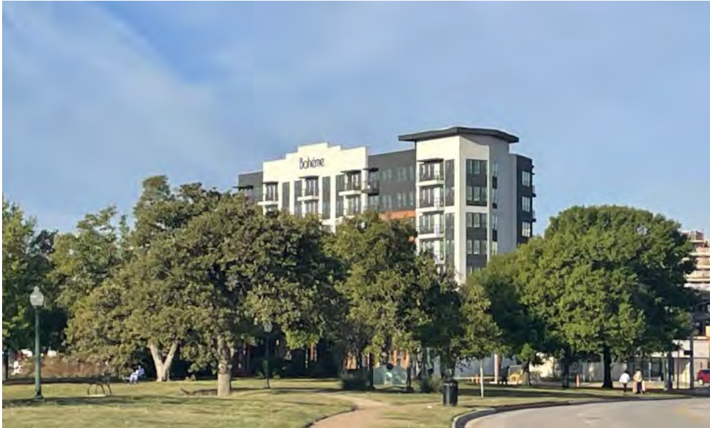
View from Lake Cliff Park looking toward the Boheme Apartments under construction at 1207 N. Zang Boulevard (formerly the site of El Fenix Restaurant).
