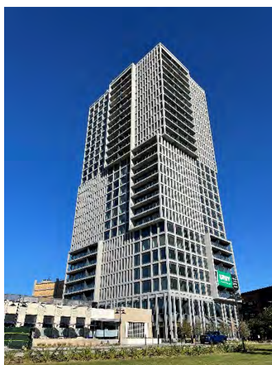
Urby Apartments Phase I nearing completion at 1930 Hi Line Drive
