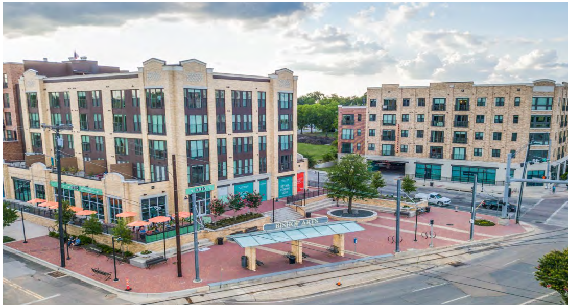
Victor Prosper Apartments (formerly known as Bishop Arts Station) with ground floor retail and a streetcar stop at the northwest corner and southwest corner of Davis Street and Zang Boulevard. Photo credit: Alamo Manhattan.
