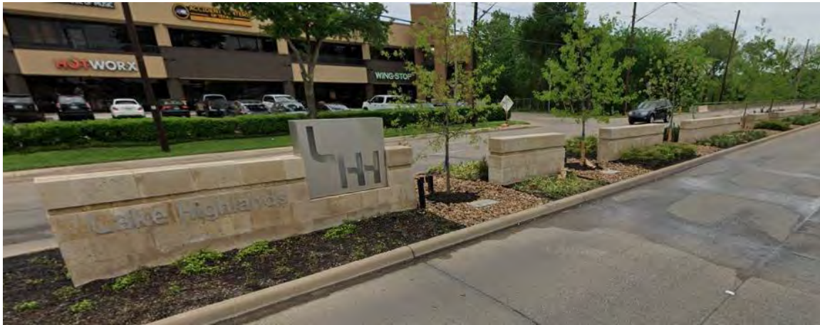
Skillman Street Median Improvements
