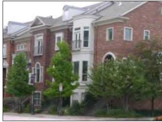
Camden Phase II - 17 Town Homes
