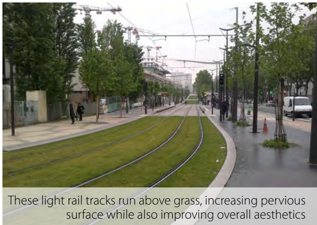
Landscaping beneath the tracks and along the tracks is preferred due to aesthetics and stormwater management
