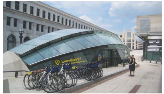
The exterior of the Washington DC Union Station METRO bike storage facility
