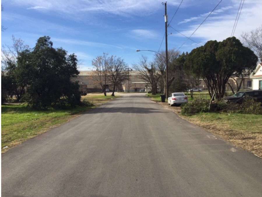
“A” Condition - New street that rides well with little to no cracks.
