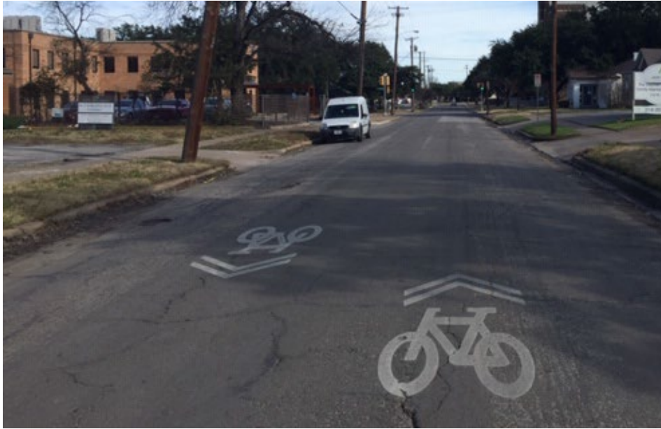
“C” Condition - Weather and Structural cracking becomes more prominent, rutting has started to develop.
