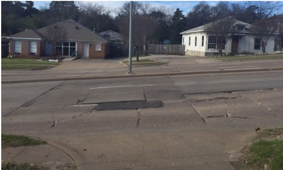
“E” Condition – Structural cracking covers over 50% of the street and frequent potholes are present.
