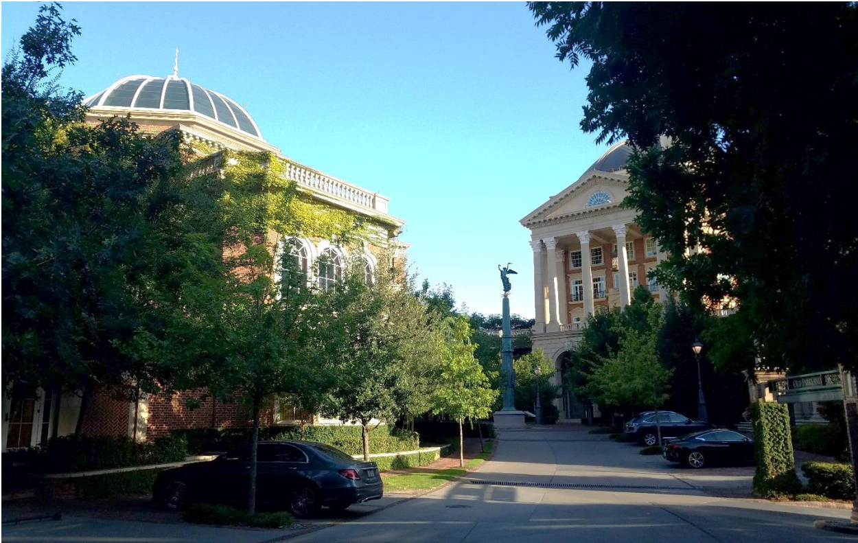
Non-Historic Structure on Campus
