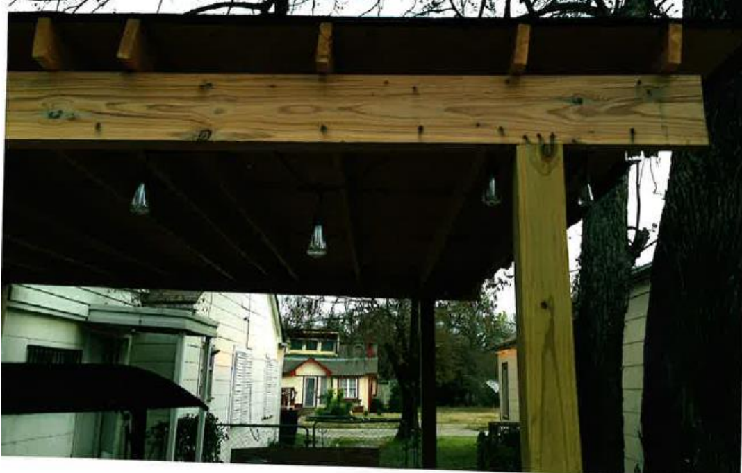
Rear porch structure. Photo submitted by applicant.
