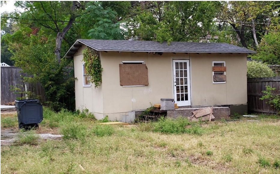
Existing siding on main and rear accessory structure
