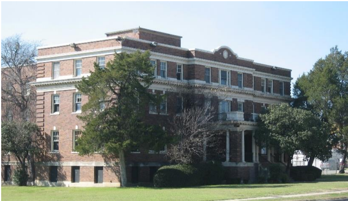
Existing Front Elevation of the Nurses Quarters Building
