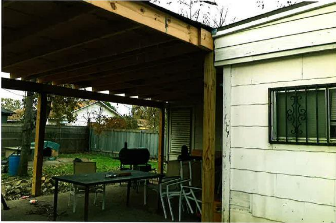
Rear porch structure. Photo submitted by applicant.
