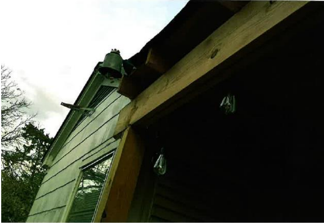
Rear porch structure. Photo submitted by applicant.
