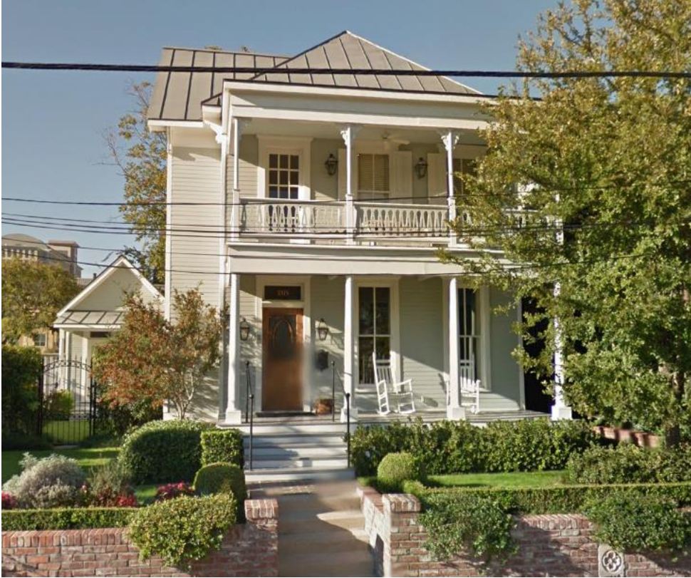
Existing Folk Victorian Structures in State Thomas – 2315 Routh St
