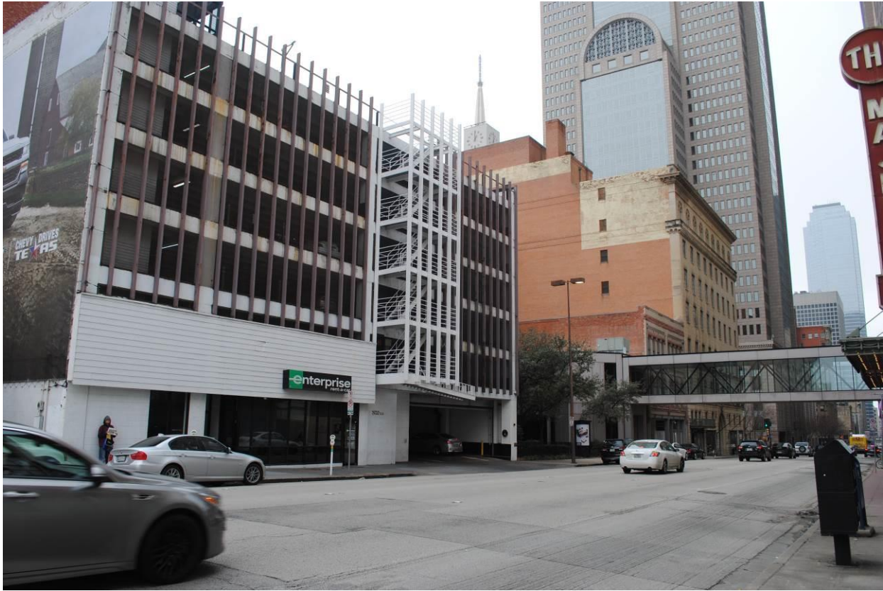
Streetscape – Facing Southwest from Elm Street (across street to the south)
