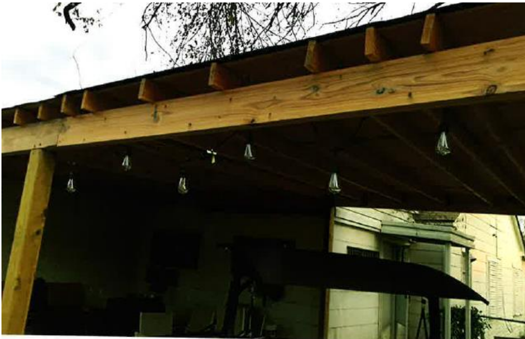
Rear porch structure. Photo submitted by applicant.
