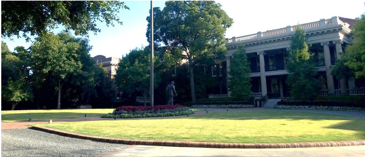
Existing Front Elevation of Old Parkland Hospital Building
