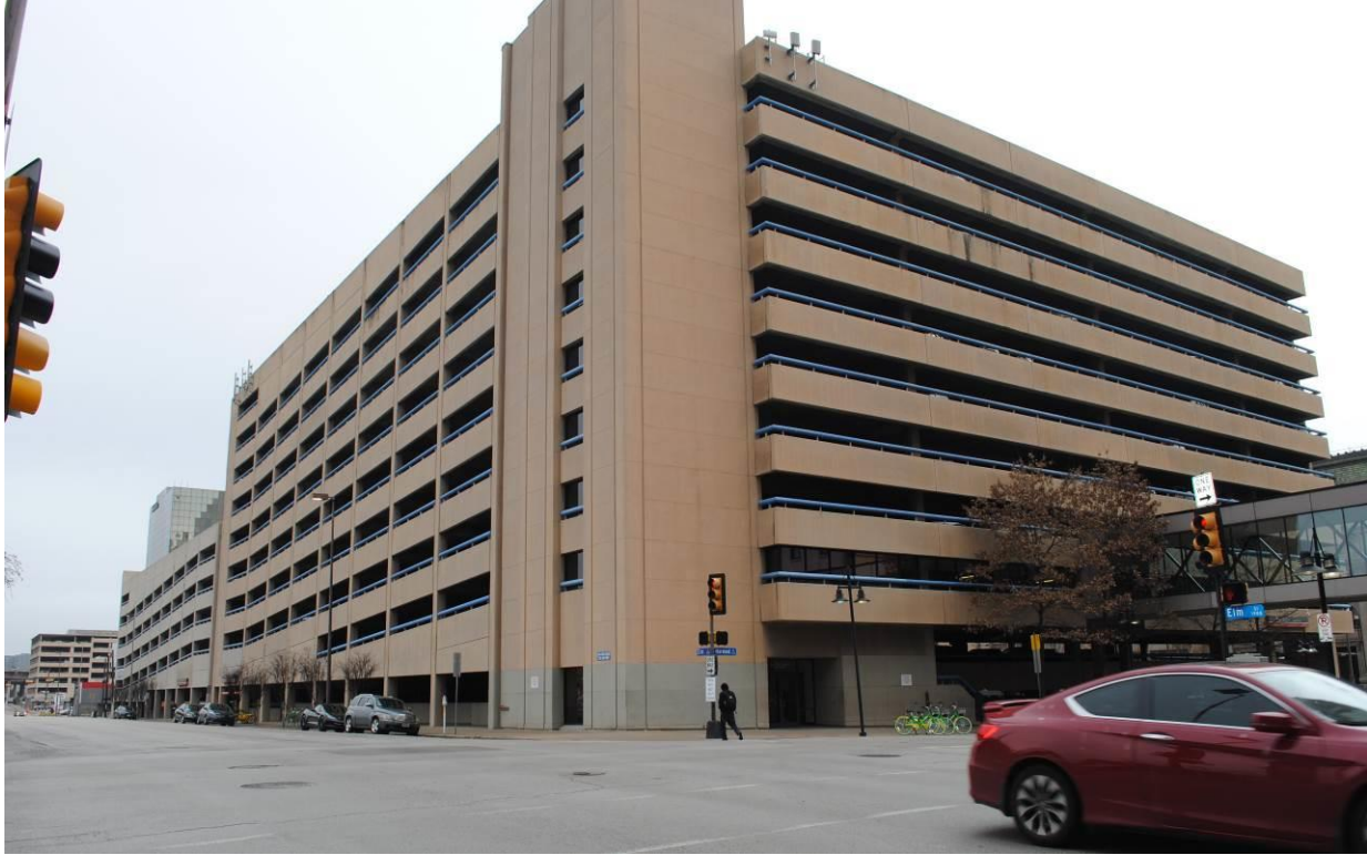
Streetscape – Facing Southeast from Elm Street (across street to the south)
