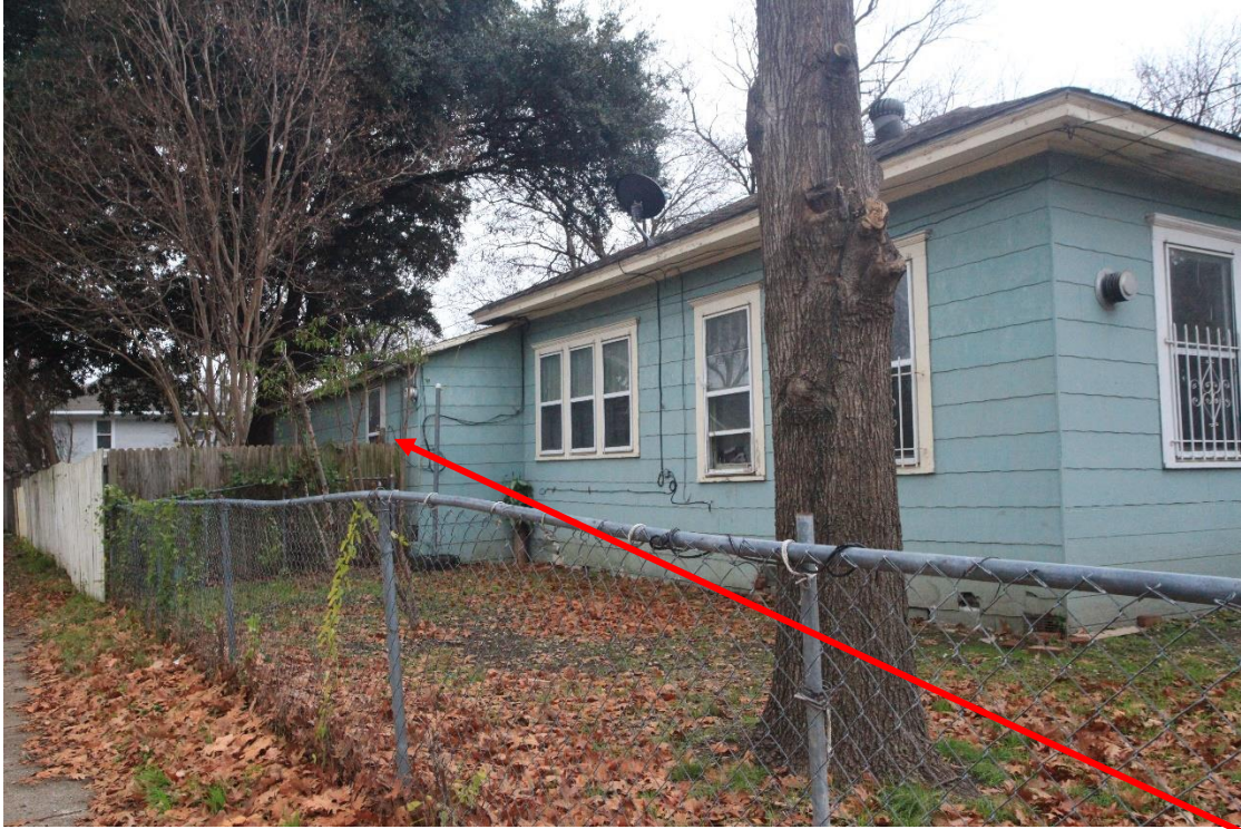
Request #2 – Corner view of left (East) side elevation with window proposed for resizing and relocation.
