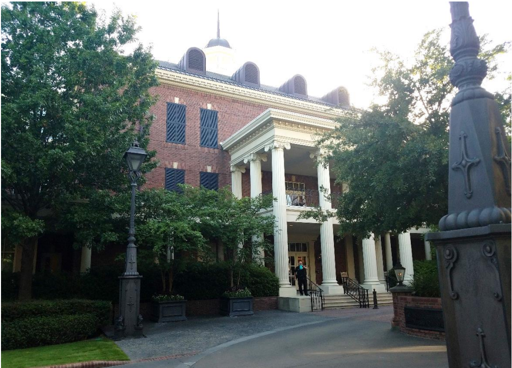
Non-Historic Structure on Campus
