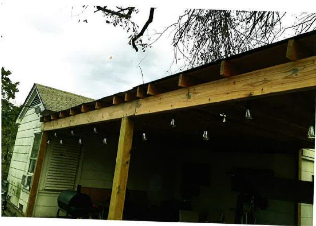
Rear porch structure. Photo submitted by applicant.
