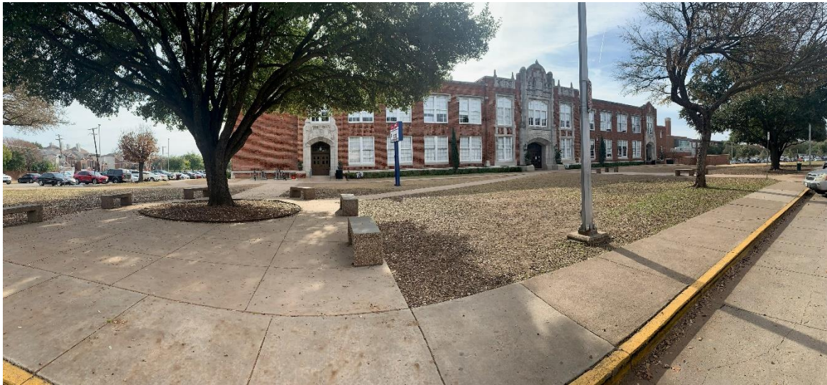
Existing West (Front) Elevation of School – Left Side of Lawn
