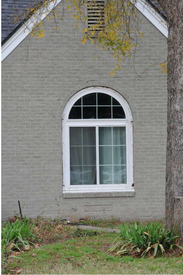
Newly installed vinyl window
