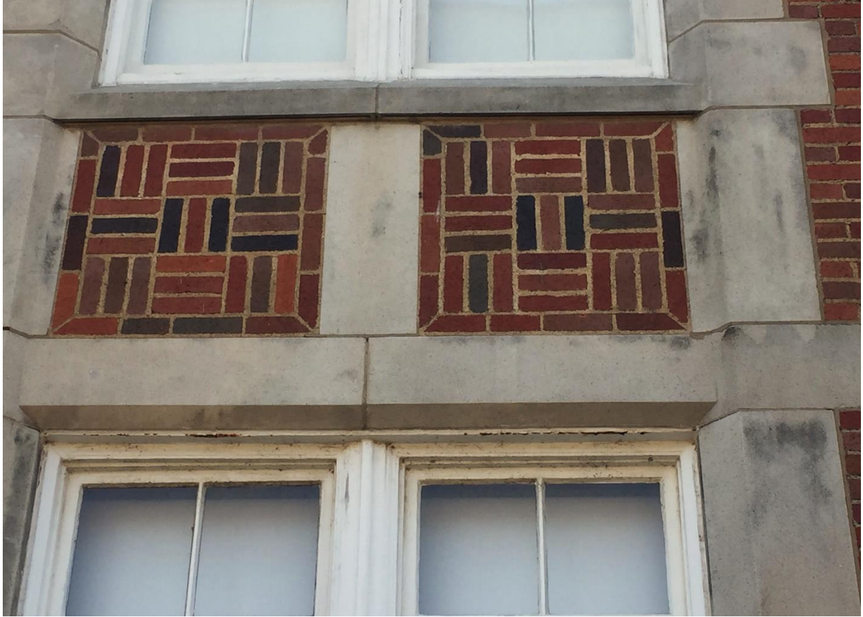
Photo of Existing Brick Exterior of School
