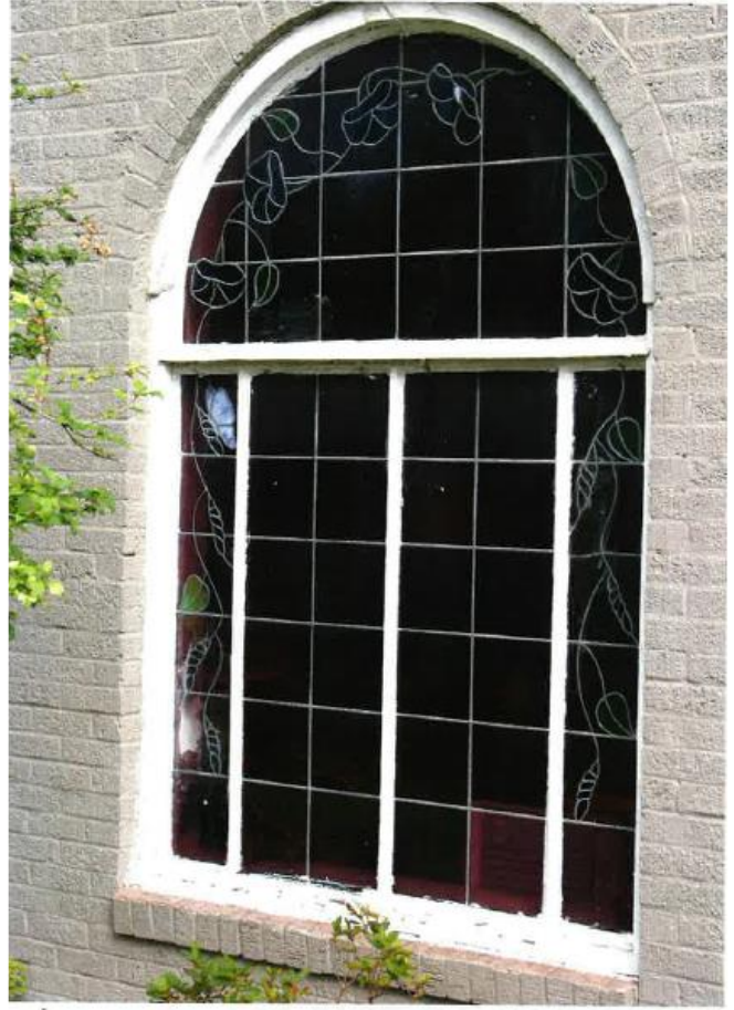
Previously existing wood window
