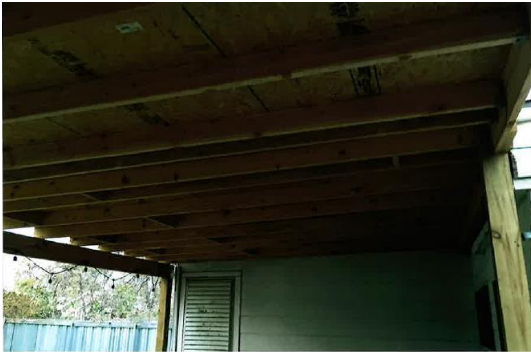
Rear porch structure. Photo submitted by applicant.
