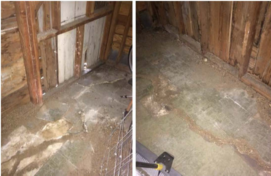
Slab foundation crack from interior; crack runs across structure sub-dividing it into two parts
