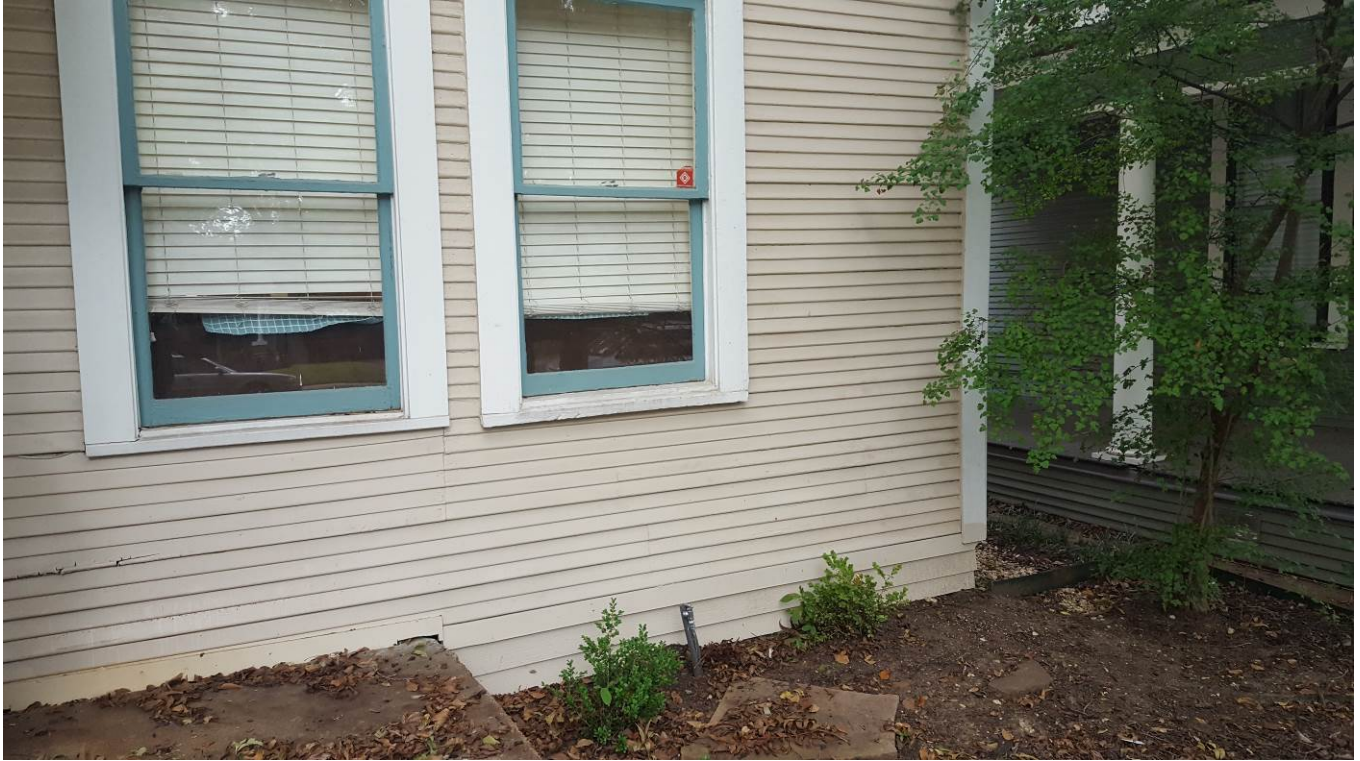
Hardiboard installed in front façade.
