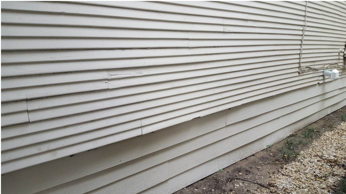
Hardiboard installed on side façade.
