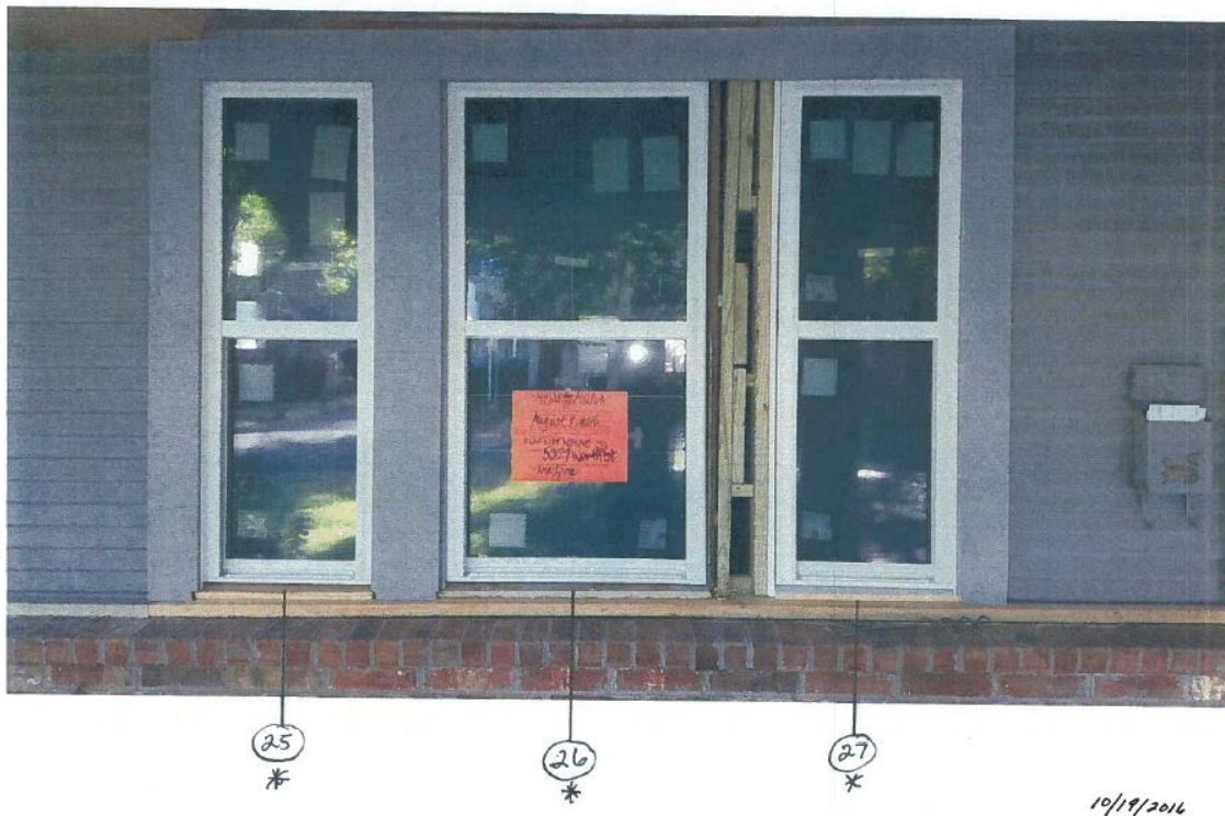
Window #s 25, 26, and 27 on front (South) elevation. Window #26 was reduced in size and Window #s 25 and 27 are newly created.
