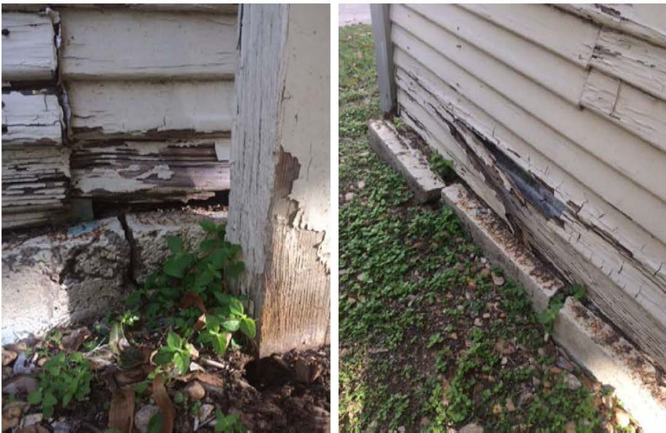
Crack at foundation wall of accessory structure near carport post, at left, and additional three cracks toward the west, at right. These exterior views are in the location of the crack that runs north-south through the entire slab, visible on the interior.
