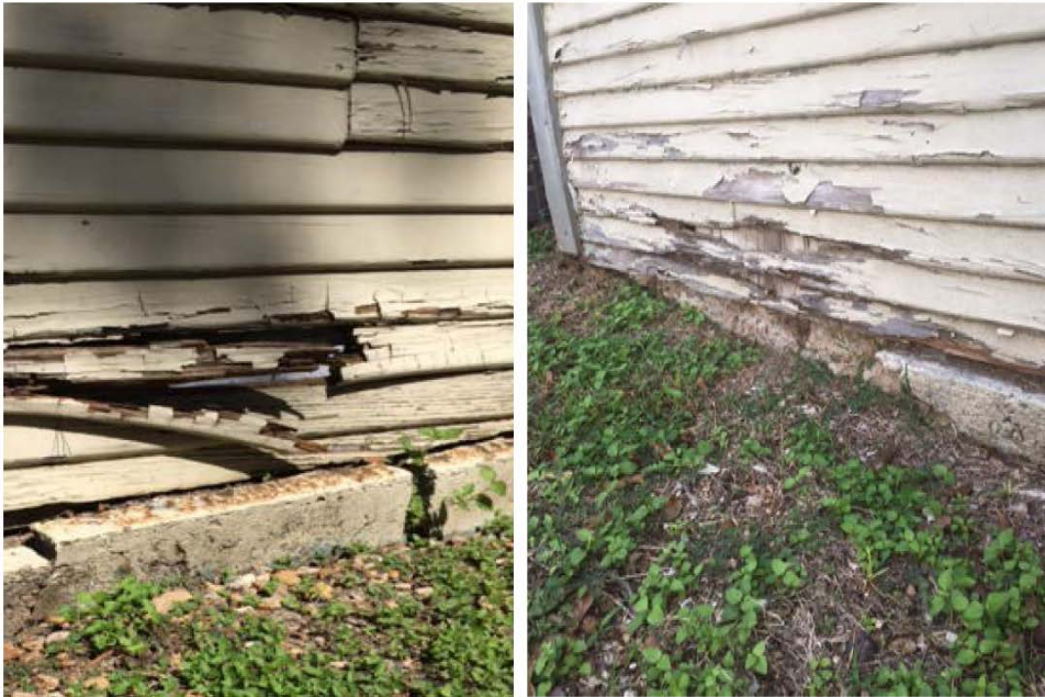
Cracked slab and poor siding conditions at south wall of accessory structure, at left, and sunken northwest corner, at right
