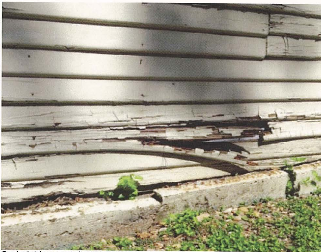
Cracked slab at servant's quarters and deteriorated siding
