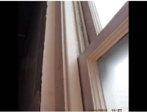
Side view of jamb w/ seam line of weight access pocket.
