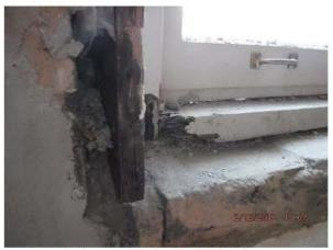
Termite damage to interior side of sill board.
