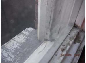
Undercut of side jamb for sill replacement (Improper repair)
