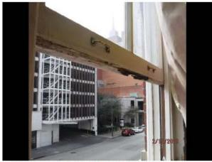
Bottom rail rot only visible when sash is raised.
