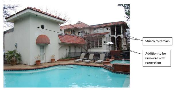
Removing the garage and roof deck and roof pavillion, which are not original to the house. Also extending the back side of the house out and adding a downstairs terrace and new roof deck above, which was already approved by Landmark Commission with CA167-100 and CA167-084.
