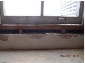
Interior blocking to give replacement sill slope to exterior.
