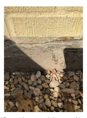
Brick after 15 minutes of Prosoco (recommended amount of time to sit so as not to dry), water and scrub brush used as well.
