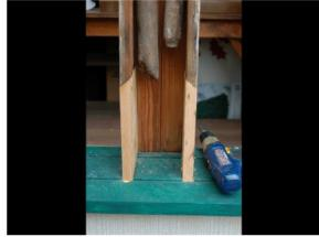
Example of Dutchman repairs to side jambs properly installed.
