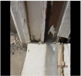
Improper sill replacement by cutting next to side jamb.
