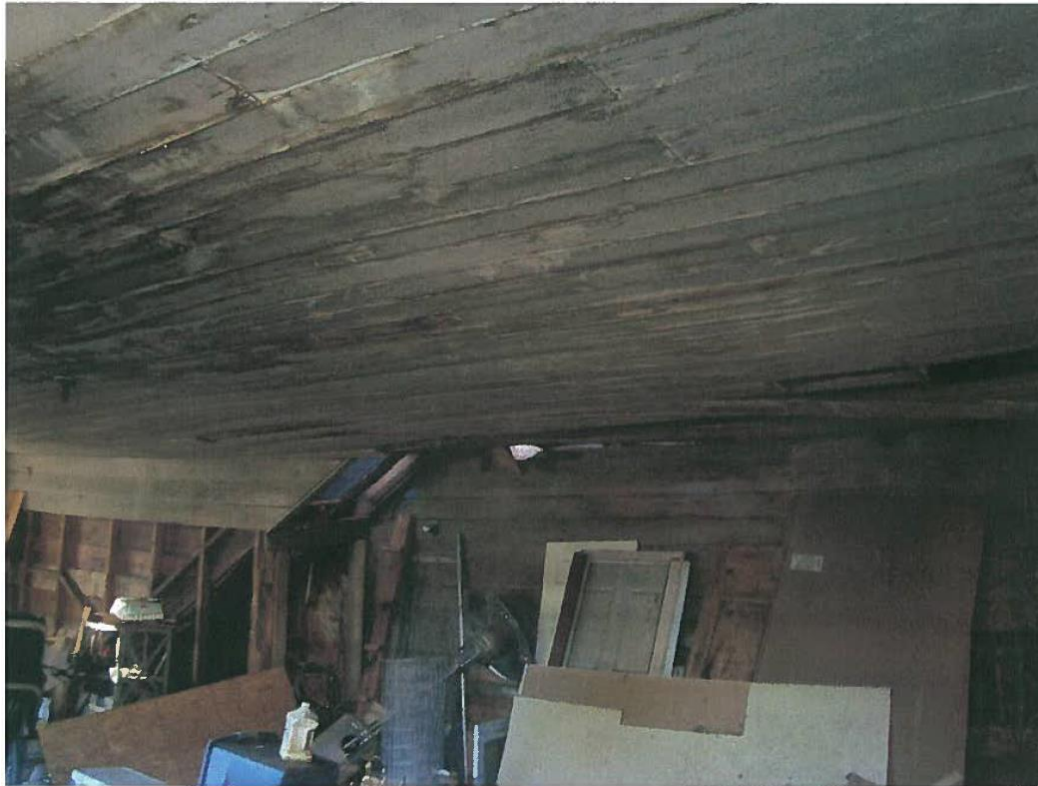
Interior showing joist failure of second floor framing.
