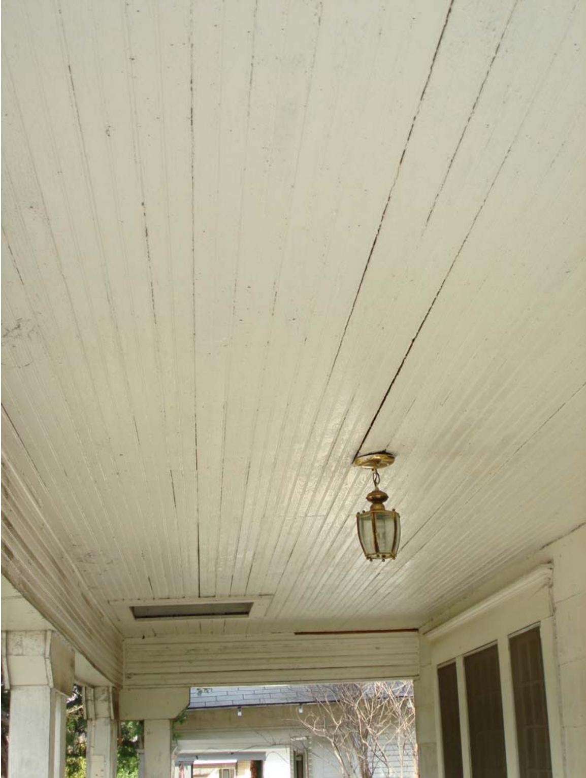
Request #3 – Existing beaded board porch ceiling.
