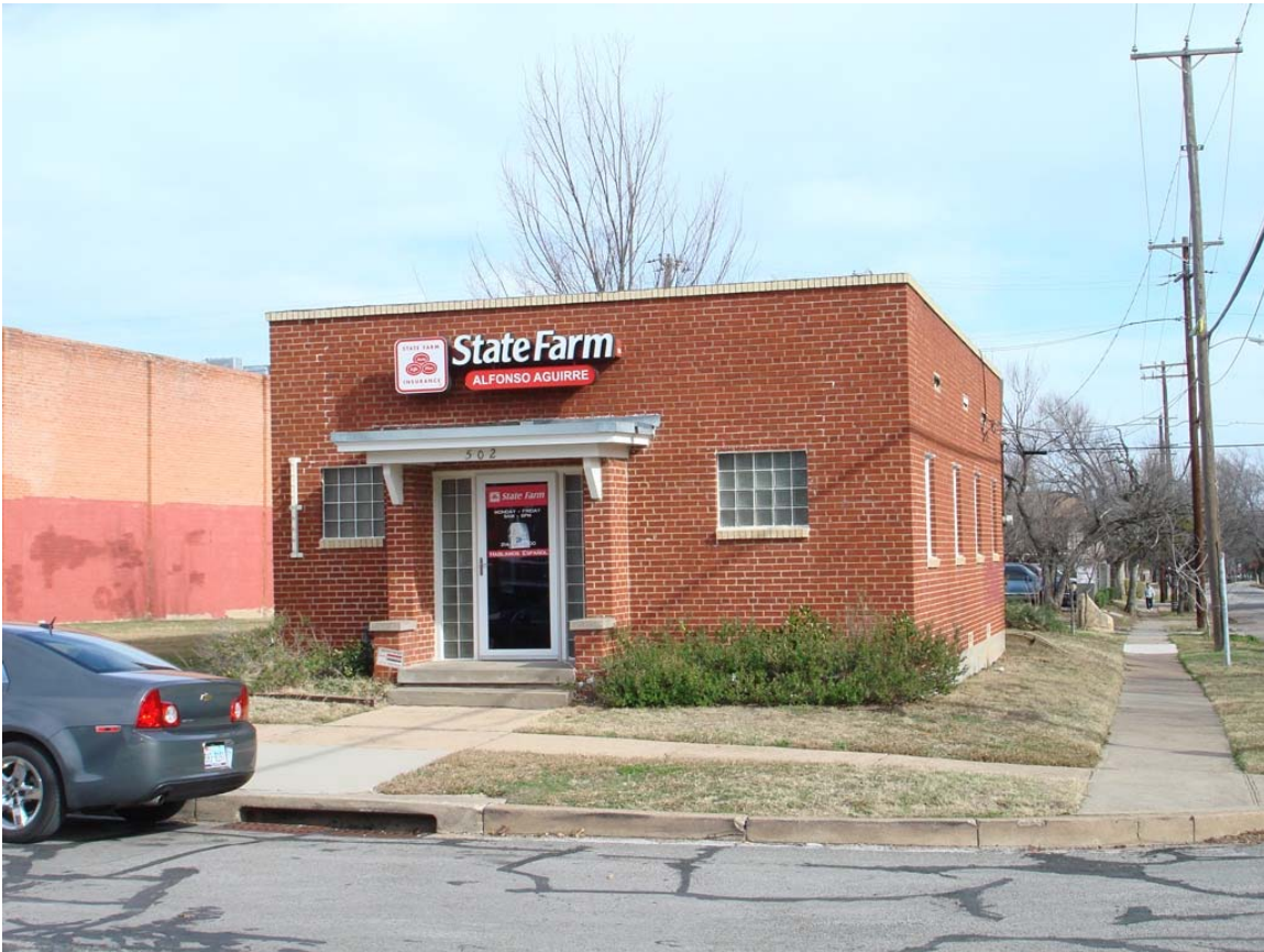
Existing signage on building.
