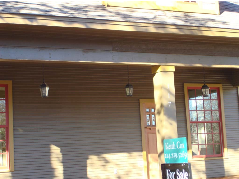
Detail of fixtures as installed.
