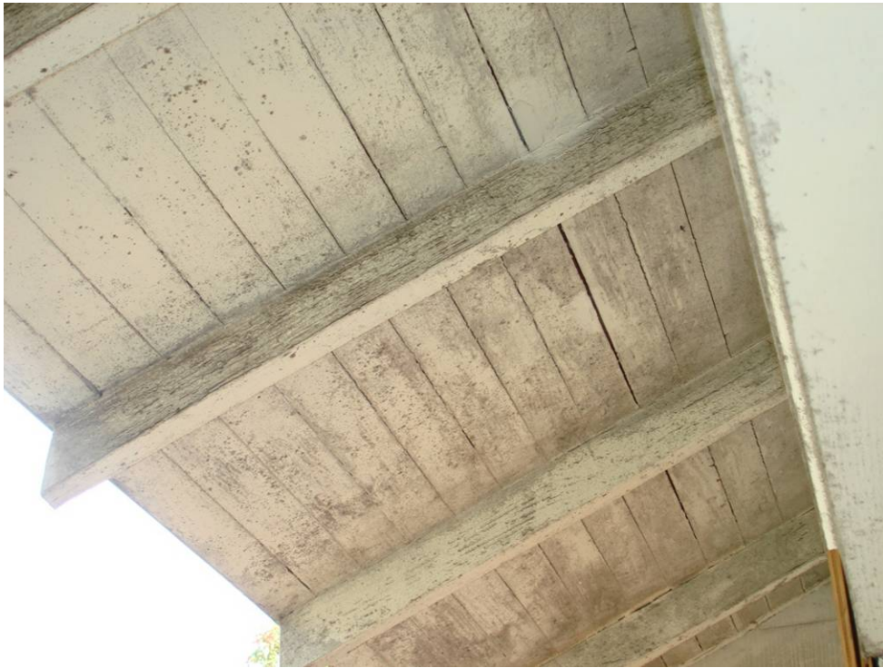
Request #1 - Existing roof decking/eave material.
