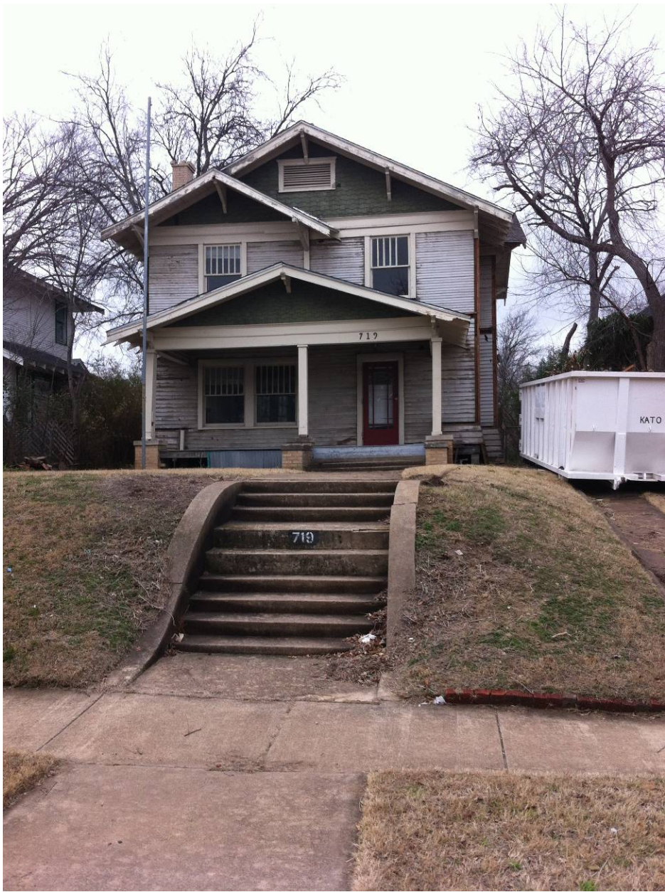
Current front facade
